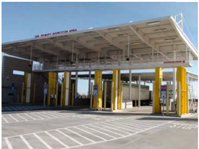
Primary Commercial Inspection Facility at the San Luis II LPOE
