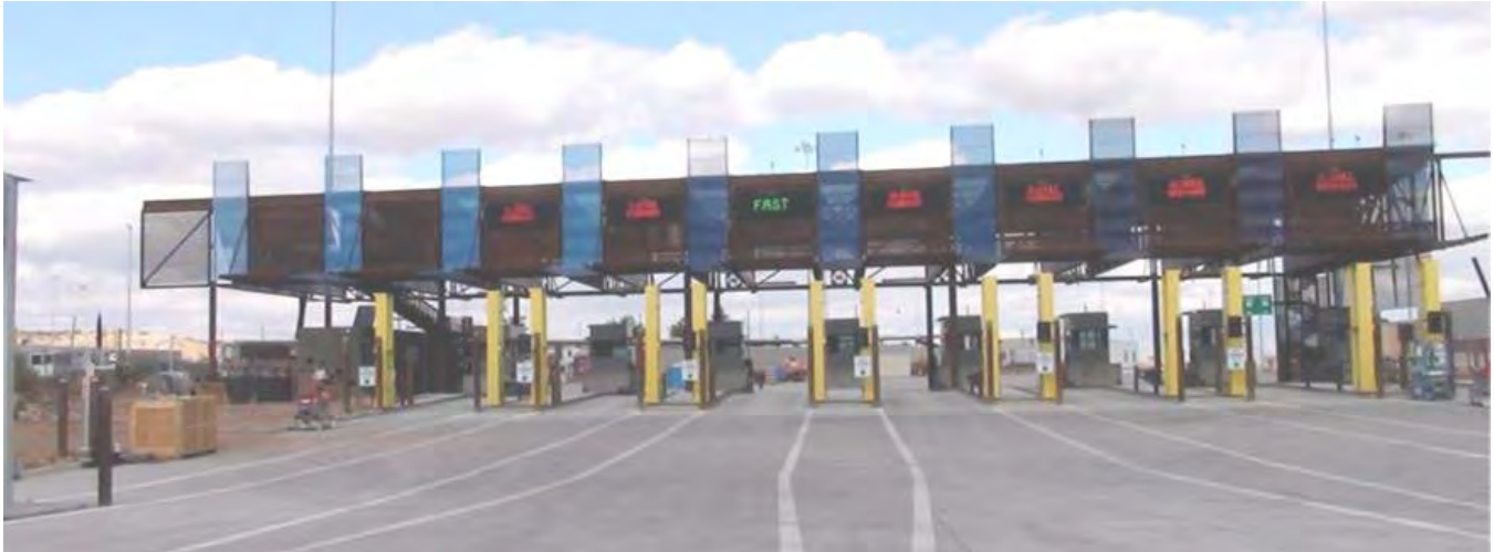
Primary Commercial Inspection Facility, Nogales Mariposa LPOE: Eight Lanes
