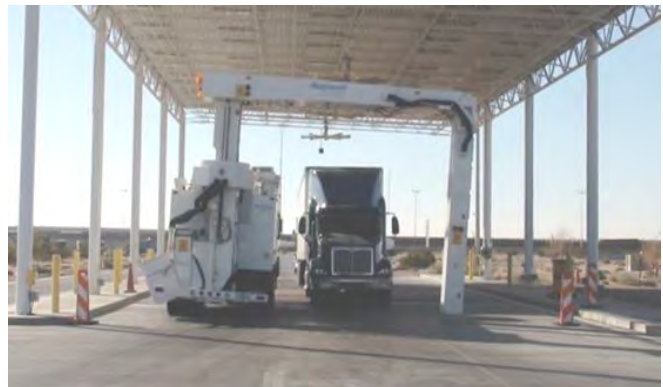
Non-Intrusive Inspection (NII) Facility at the San Luis II LPOE
