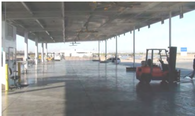
Secondary Commercial Inspection Facilities – Docks at the San Luis II LPOE
