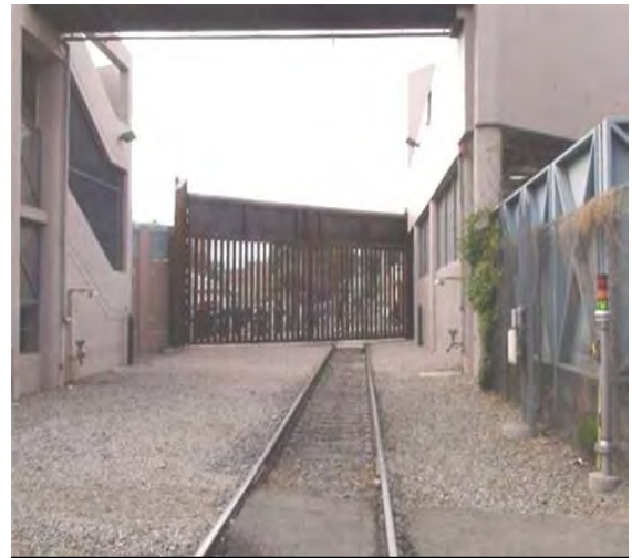
Border Rail Gates at DeConcini LPOE
