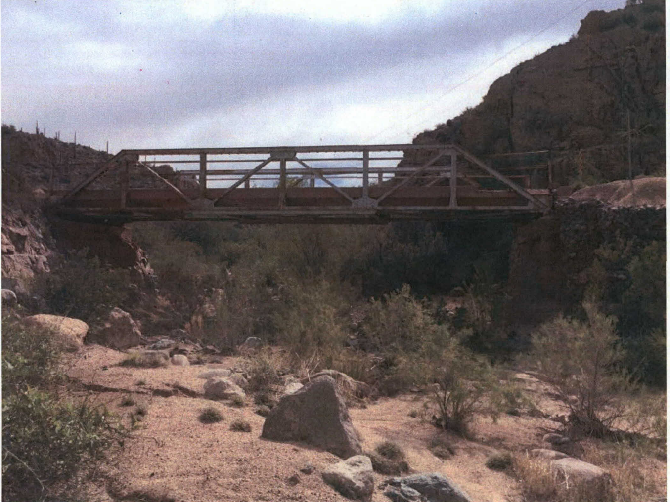
File Name : 00028-2018-08-30-Photo-C.jpg Description : Photo C - Elevation ID looking East
