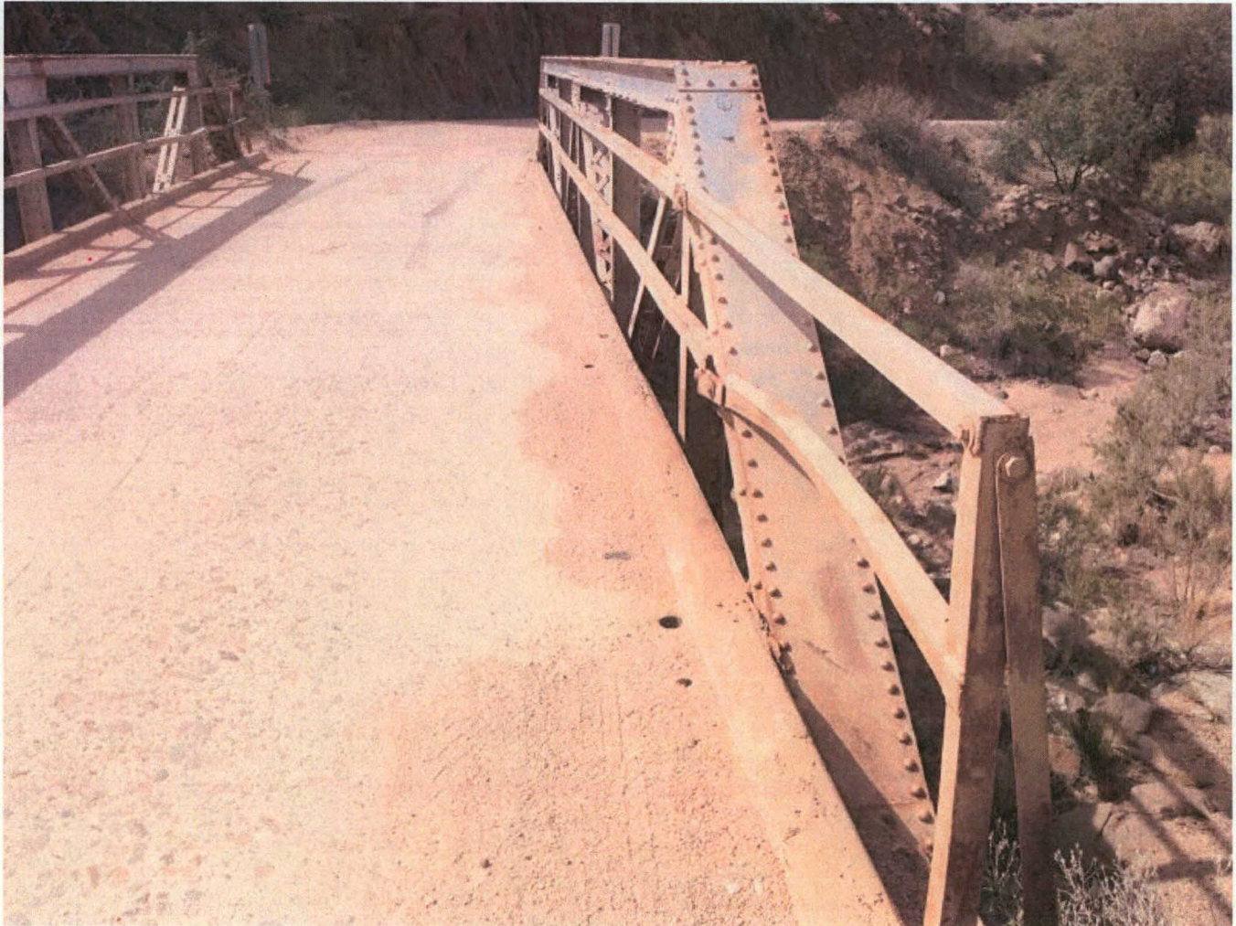
File Name : 00028-2018-08-30-Photo-K.jpg Description : Photo K – West Truss looking South
