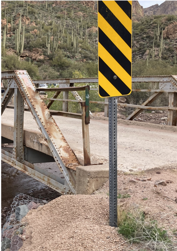
Figure 3: Existing Conditions at Lewis Pranty Creek Bridge
