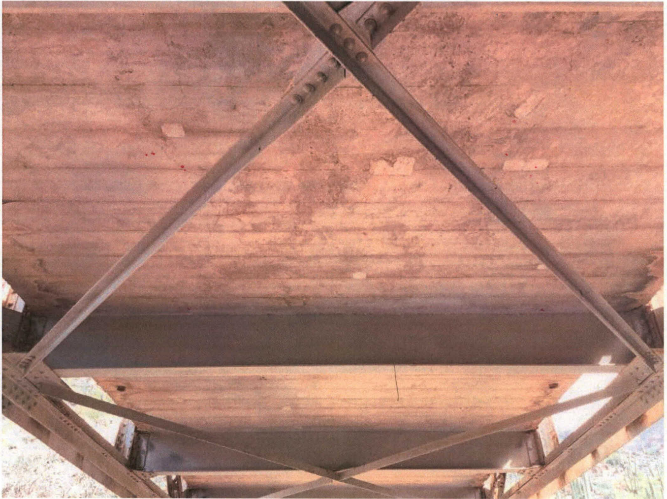
File Name : 00028-2018-08-30-Photo-I.jpg Description : Photo I – Typical Bottom of Deck
