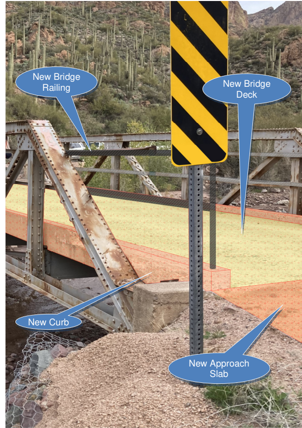
Figure 4: Proposed Improvements at Lewis Pranty Creek Bridge
