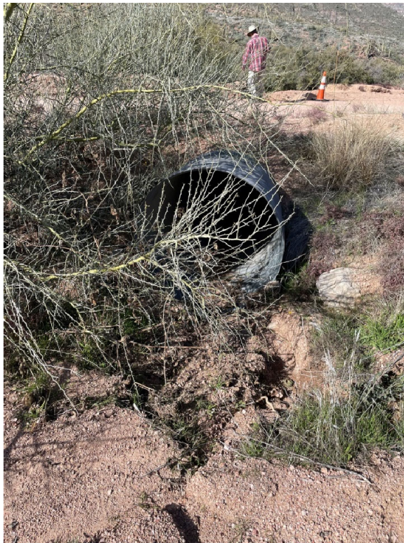
Existing upstream end of CMP at approximately MP 228
