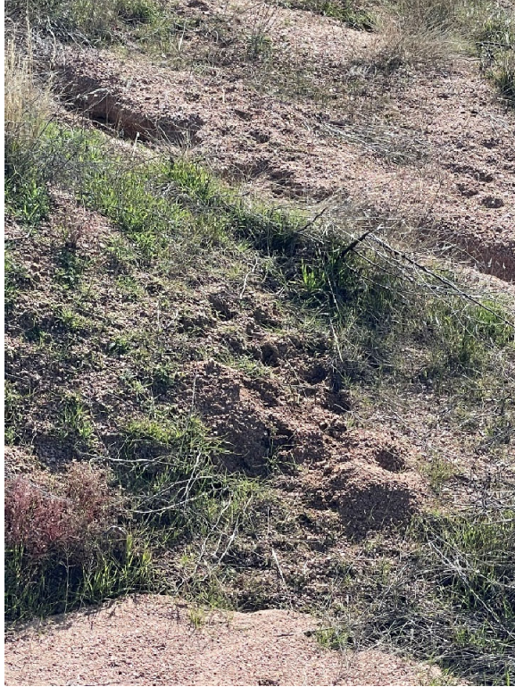
Buried inlet at east end of project
