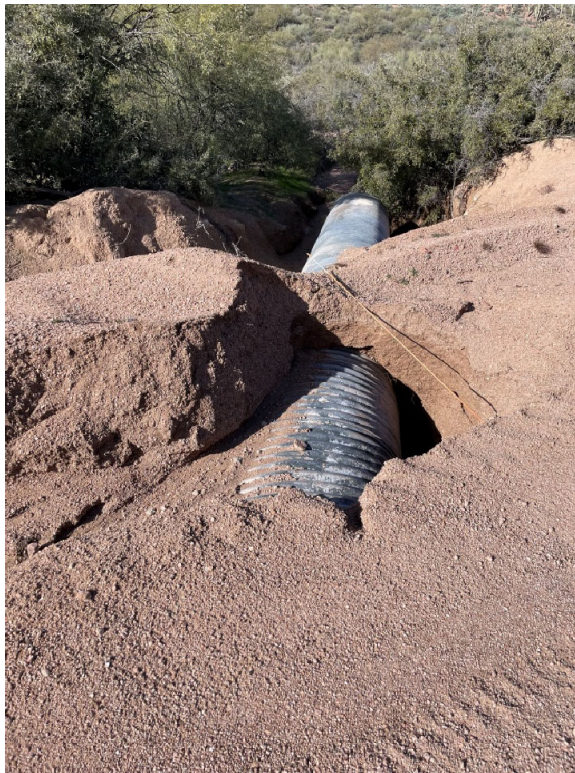
Existing downstream end of CMP at approximately MP 228
