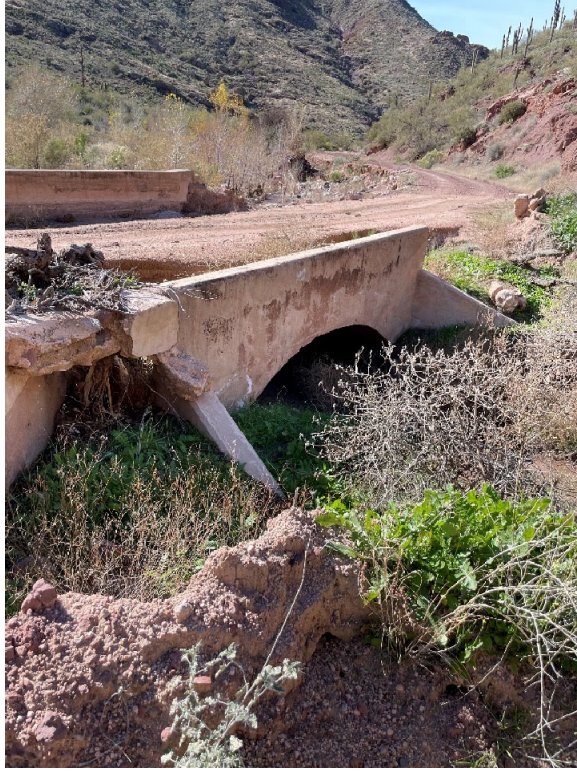
Inlet of Culvert at approximately MP 225.8
