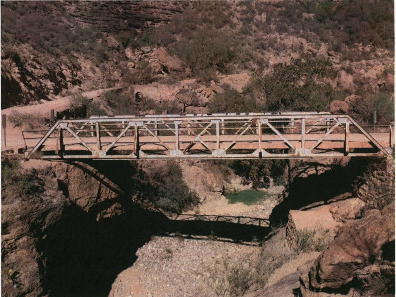
File Name : 00027-2018-09-08-Photo-B.jpg Description : Photo B. Elevation ID, looking West
