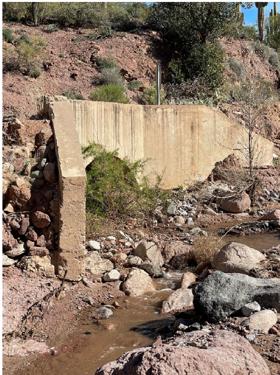
Outlet of culvert at approximately MP 225.8
