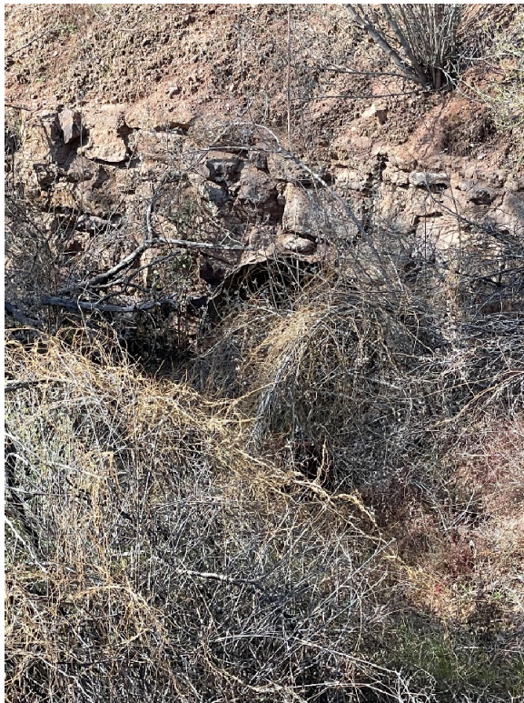
Existing culvert outlet at east end of project
