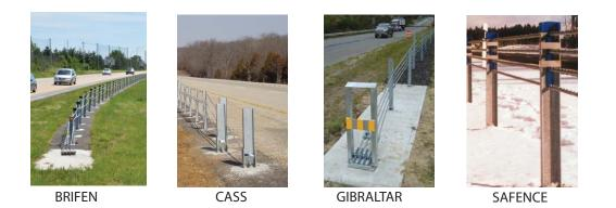
Like all barriers, it is important to properly design, install, and maintain HTCB for the best performance. To function properly in an impact, a HTCB must be able to gradually redirect or arrest an impacting vehicle by cable deflection, which minimizes forces on the vehicle and its occupants. To obtain the desired results, the cables must be properly tensioned and at the correct heights above the ground.
