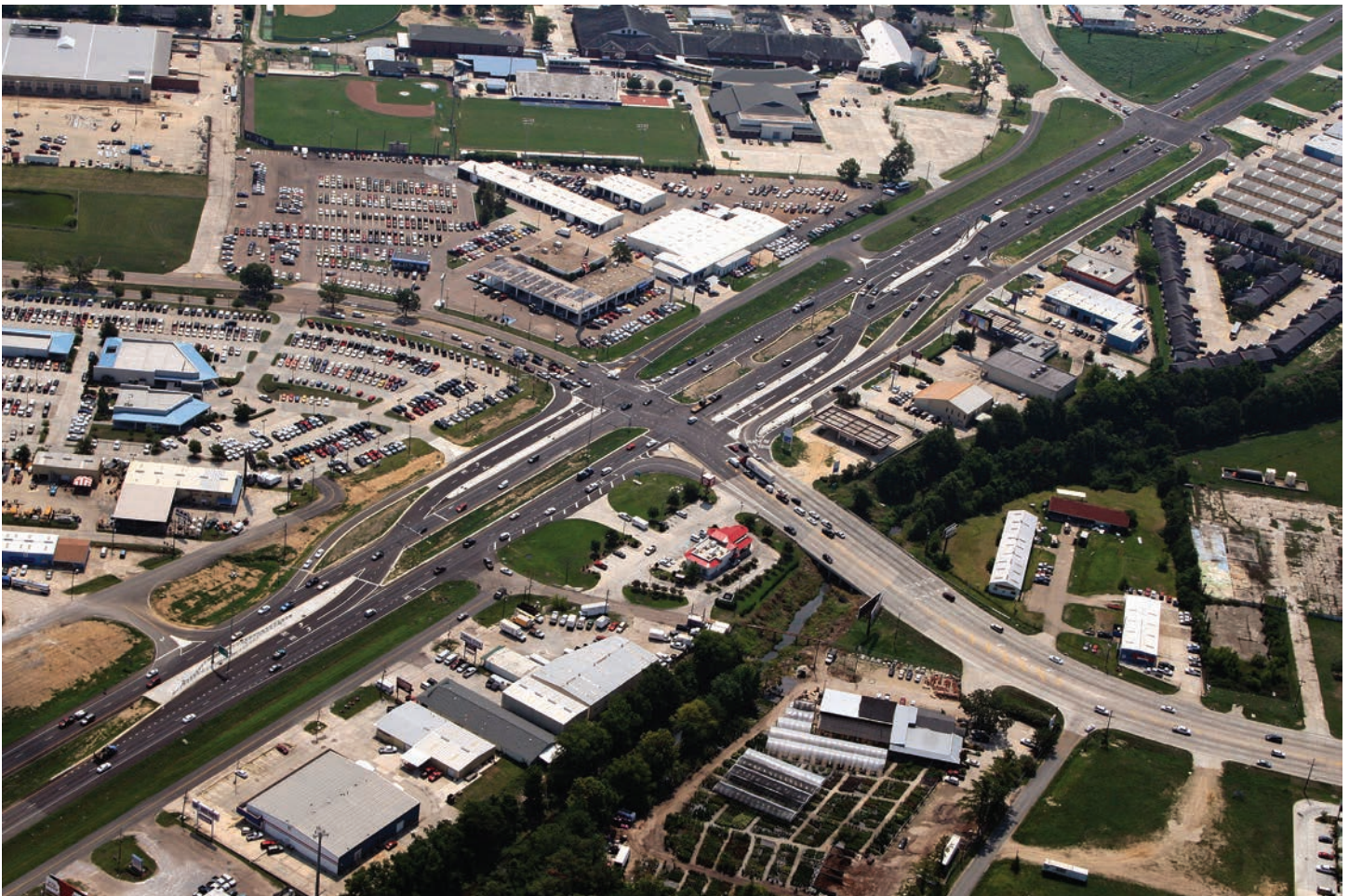
Airline Highway Continuous Flow Intersection
