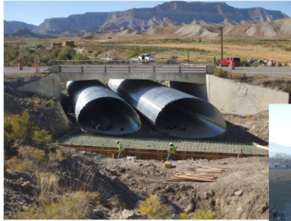
Twin cell 18'-7" x 12' Structural Plate Pipe Arch with 60 degree skew.
