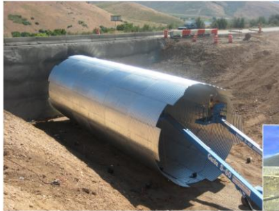
22' diameter Structural Plate with bevel cut ends and natural bottom to be used as a deer crossing
