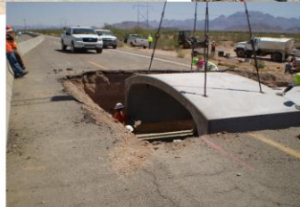
24' Concrete Arch with precast slab foundation
