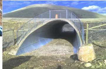
22' diameter Structural Plate with bevel cut ends and natural bottom to be used as a deer crossing
