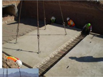
24' Concrete Arch with precast slab foundation
