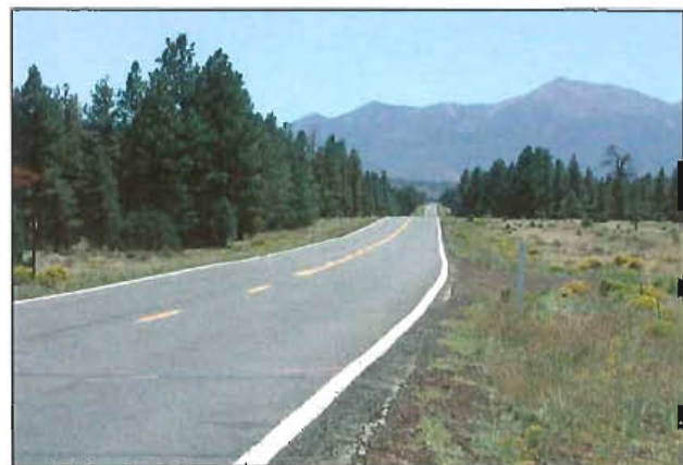
Typical view of US 180 roadway, southbound near boundary that separates Coconino and Kaibab national forests.
