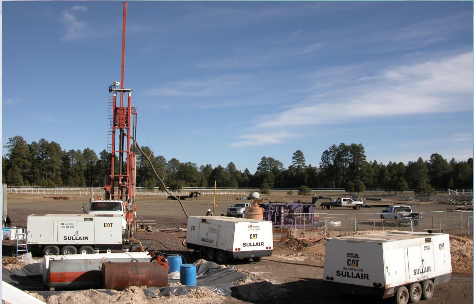
Fort Tuthill Well Dual Rotary Drilling
