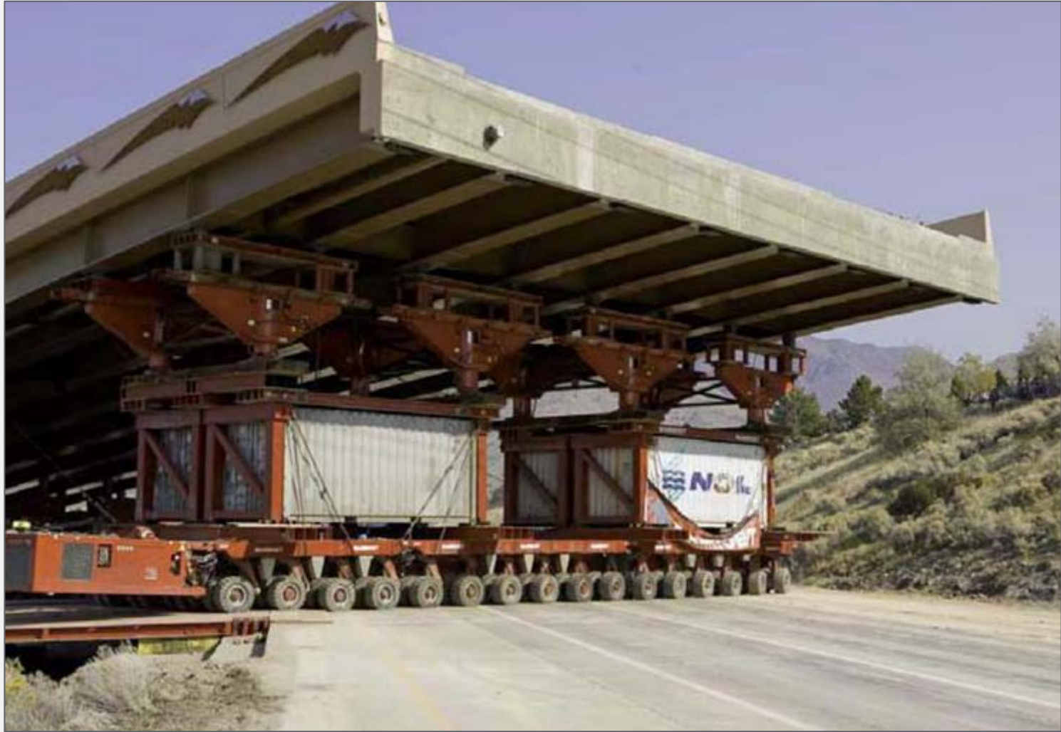
4500 SOUTH - UDOT'S FIRST ABC SPMT PROJECT - CMGC DELIVERY
