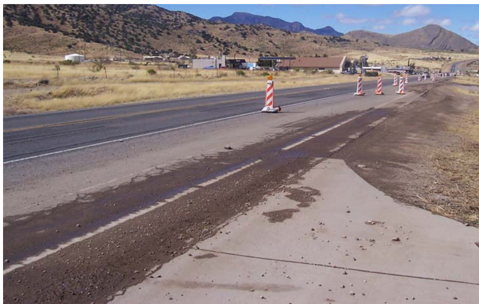
Figure 7-15. SR 92 roadside watered for dust suppression.
