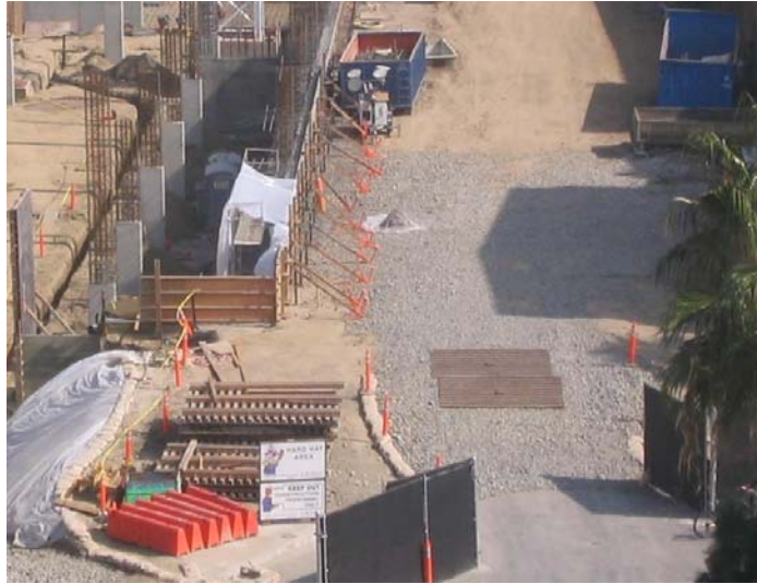
Figure A-3. Example gravel pad and “grizzly” (grate) at construction site entrance.
