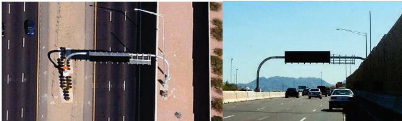
Figure 11 - Example of Difficult Maintenance Access due to Physical Barrier
