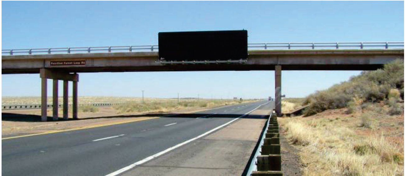
Figure 15 - Example of Rural Overhead DMS Mounted on Bridge Structure
