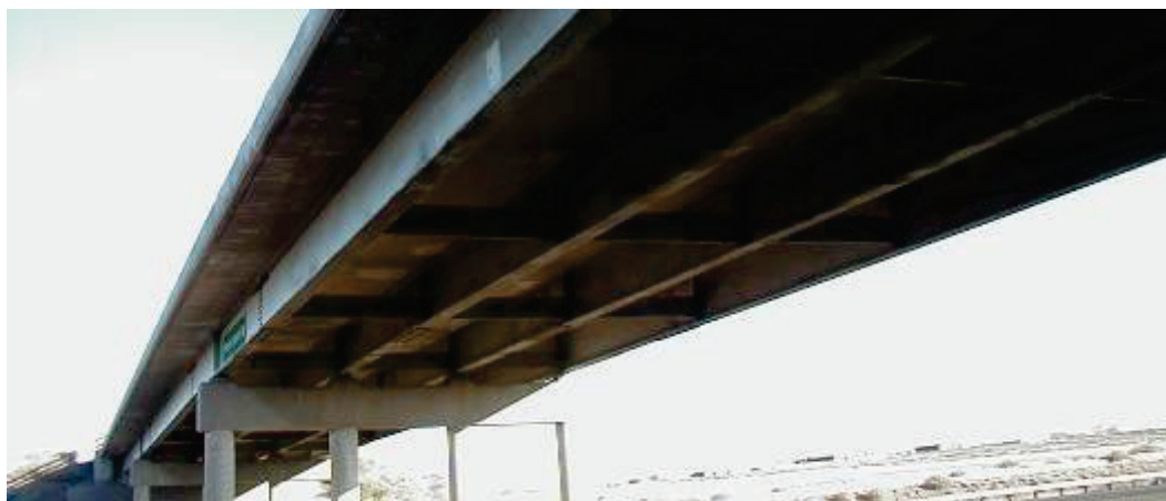
Figure 13 - Example of "Open" Bridge Structure
