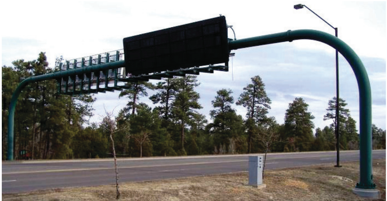
Figure 14 - Example of Opposing DMS Mounted on Same Structure (SD 9.51)
