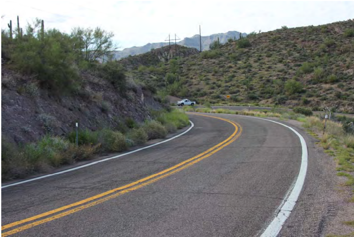
Photo 5. View to the southeast from the middle of Curve 2 at MP 204.3.
