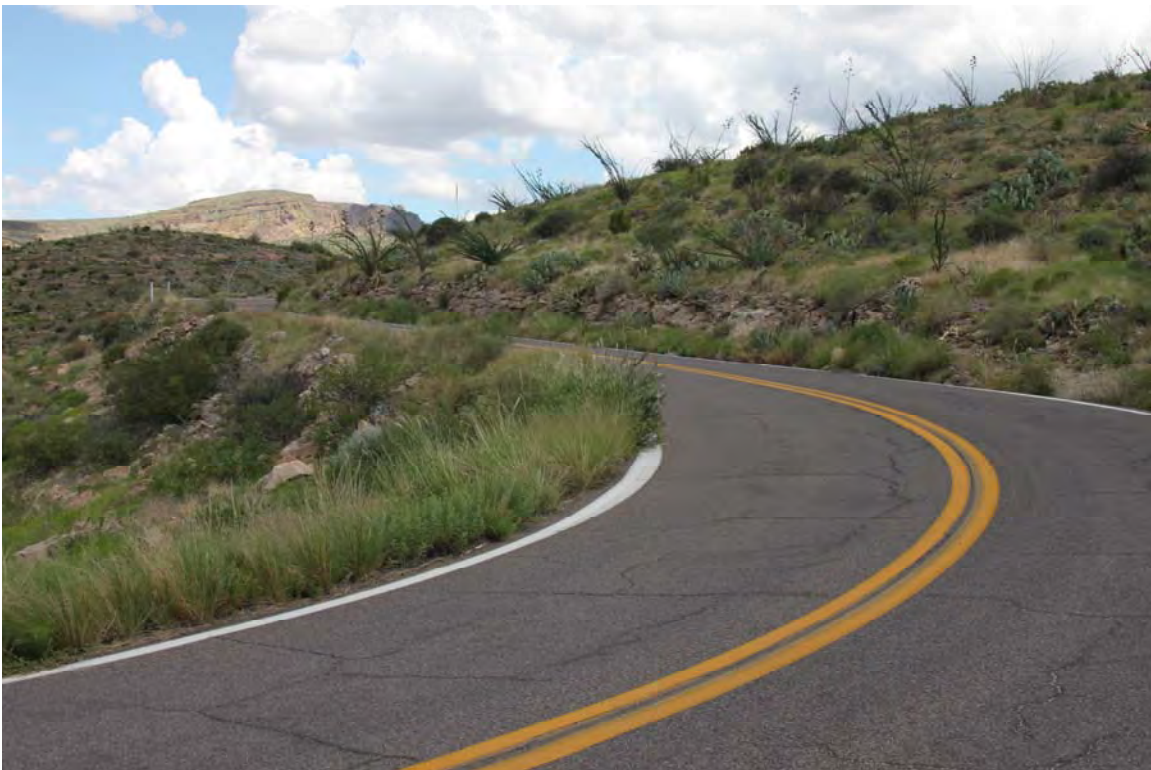
Photo 52. View to the northeast at MP 219.7 (panned right from the previous photo).
