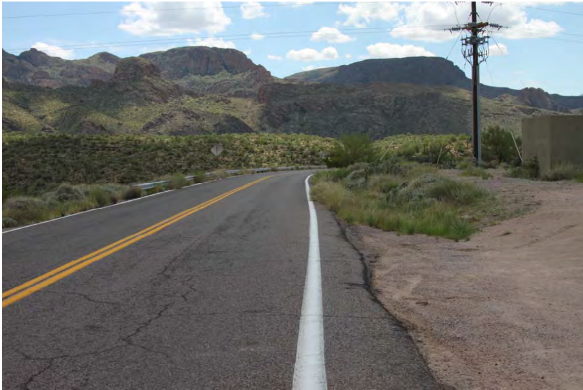
Photo 47. View to the southwest at MP 216.4.
