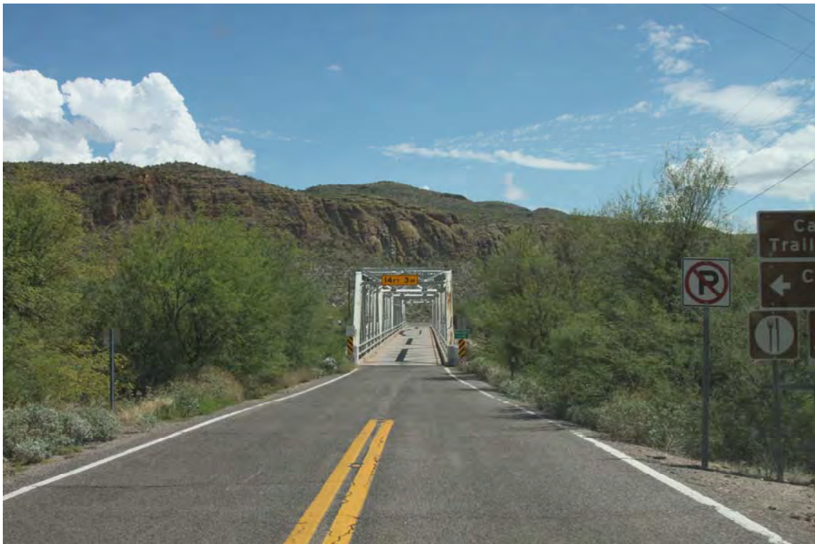
Photo 26. View to the northeast of the eastbound approach to the Boulder Canyon Bridge at MP 211.
