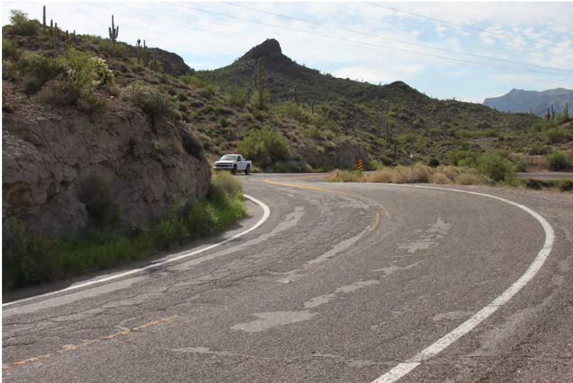
Photo 7. View to the southeast from the middle of Curve 3 at MP 204.5.
