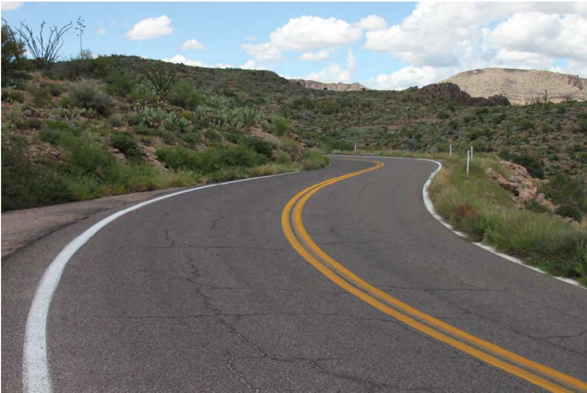
Photo 51. View to the northwest at MP 219.7.
