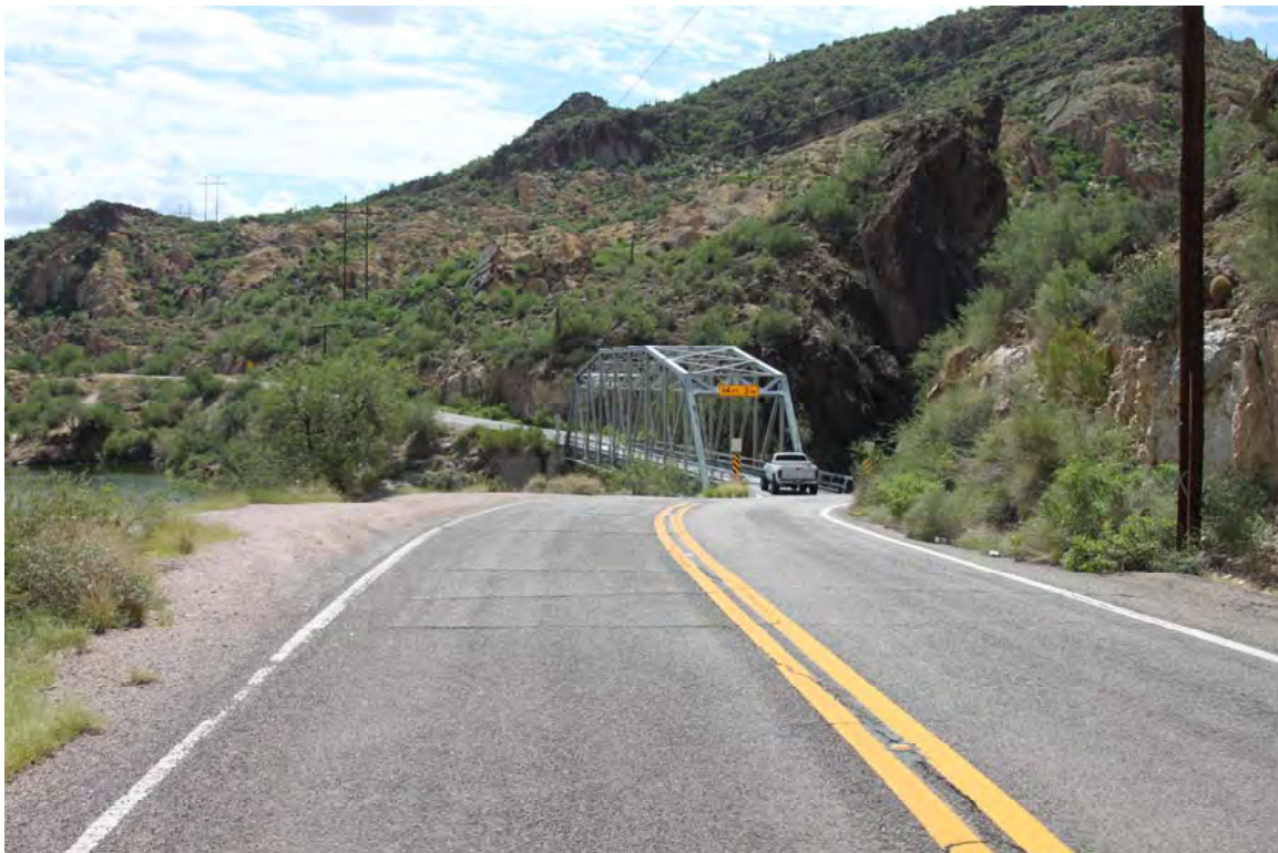
Photo 20. View to the east of the First Water Creek Bridge (Structure No. 26) at MP 209.6.
