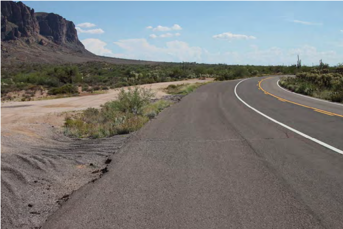
Photo 1. View to the southwest of a planned staging area at MP 201.95.
