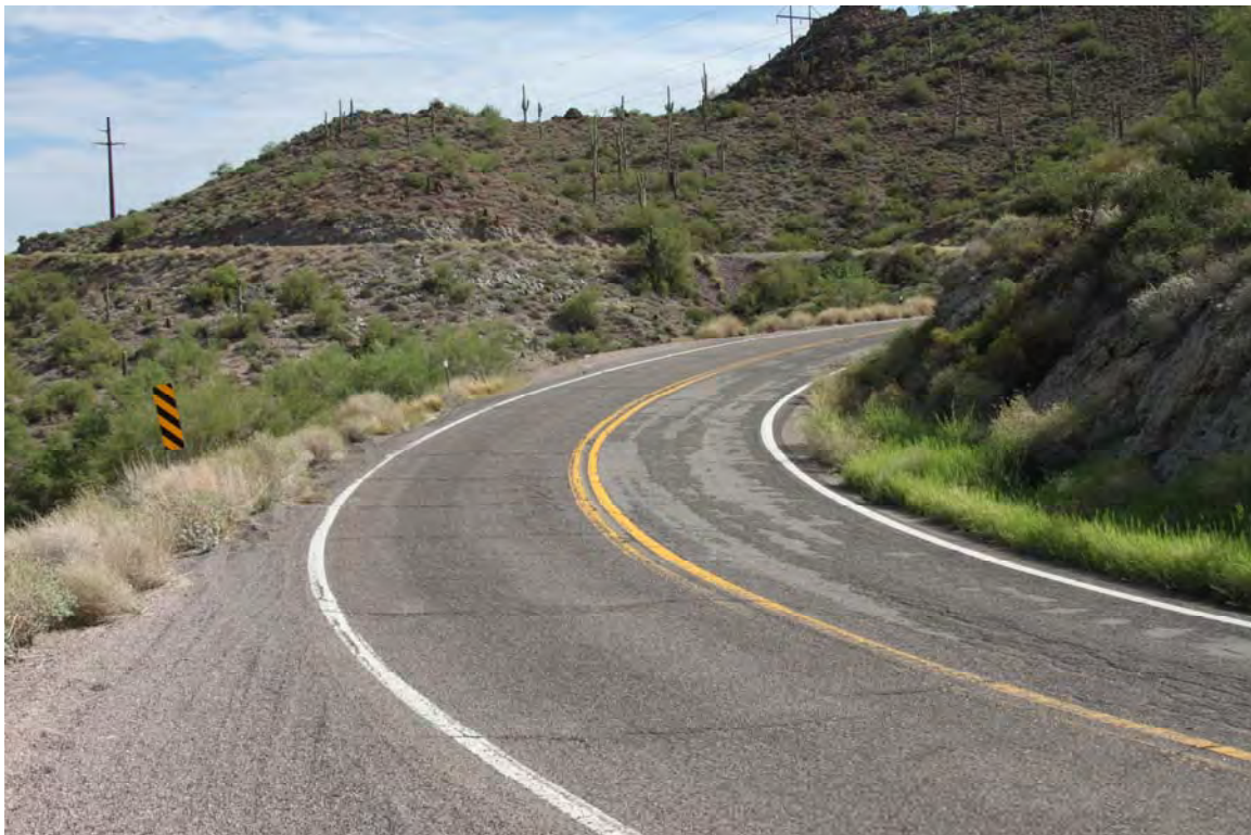
Photo 8. View to the northeast from the middle of Curve 3 at MP 204.5 (opposite view from the previous photo).
