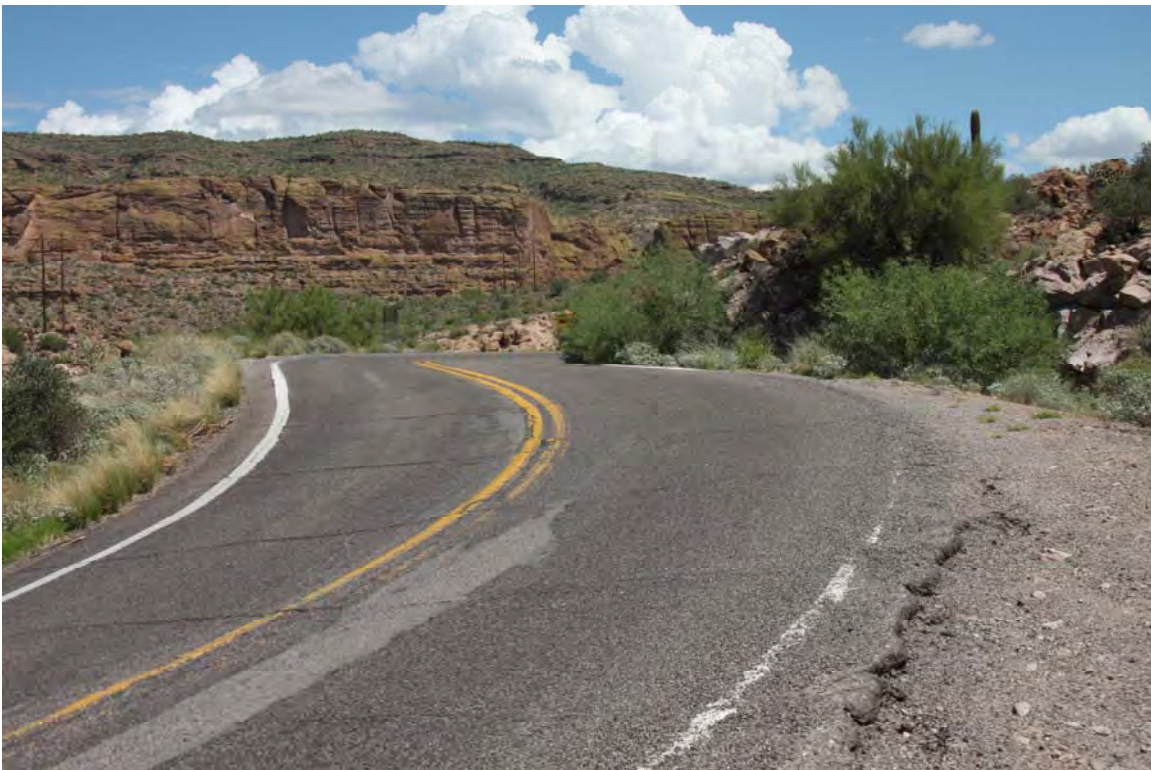
Photo 30. View to the northeast from just east of MP 212 (opposite view of the previous photo).
