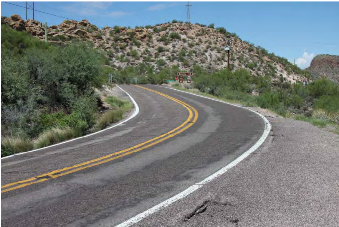
Photo 24. View to the west from the middle of Curve 6 at MP 210.45.
