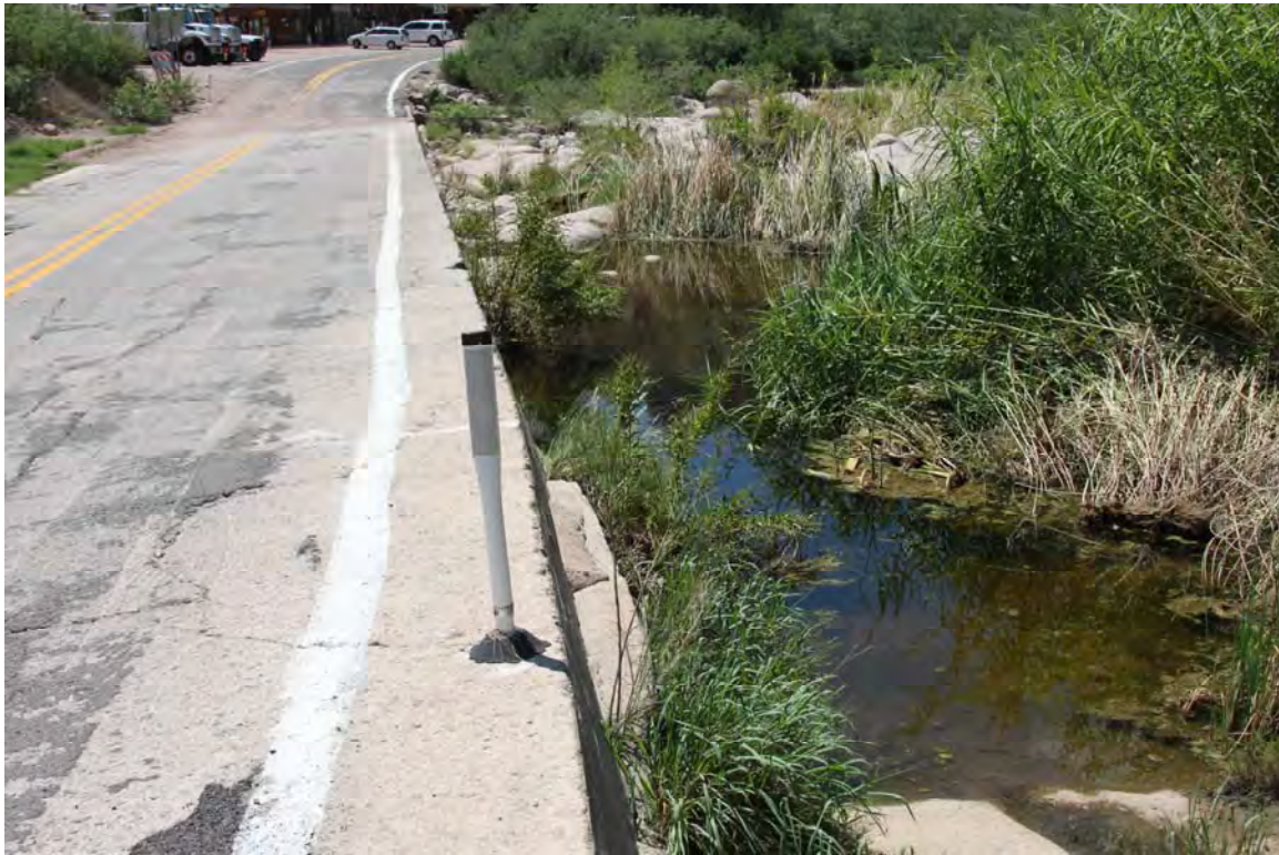
Photo 37. View to the west along the downstream (north) side of the ford crossing of Tortilla Creek.
