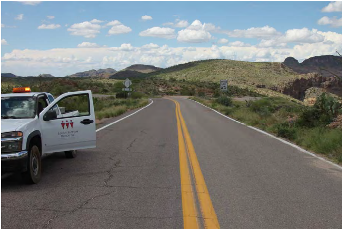
Photo 53. View to the northwest at MP 220.2.
