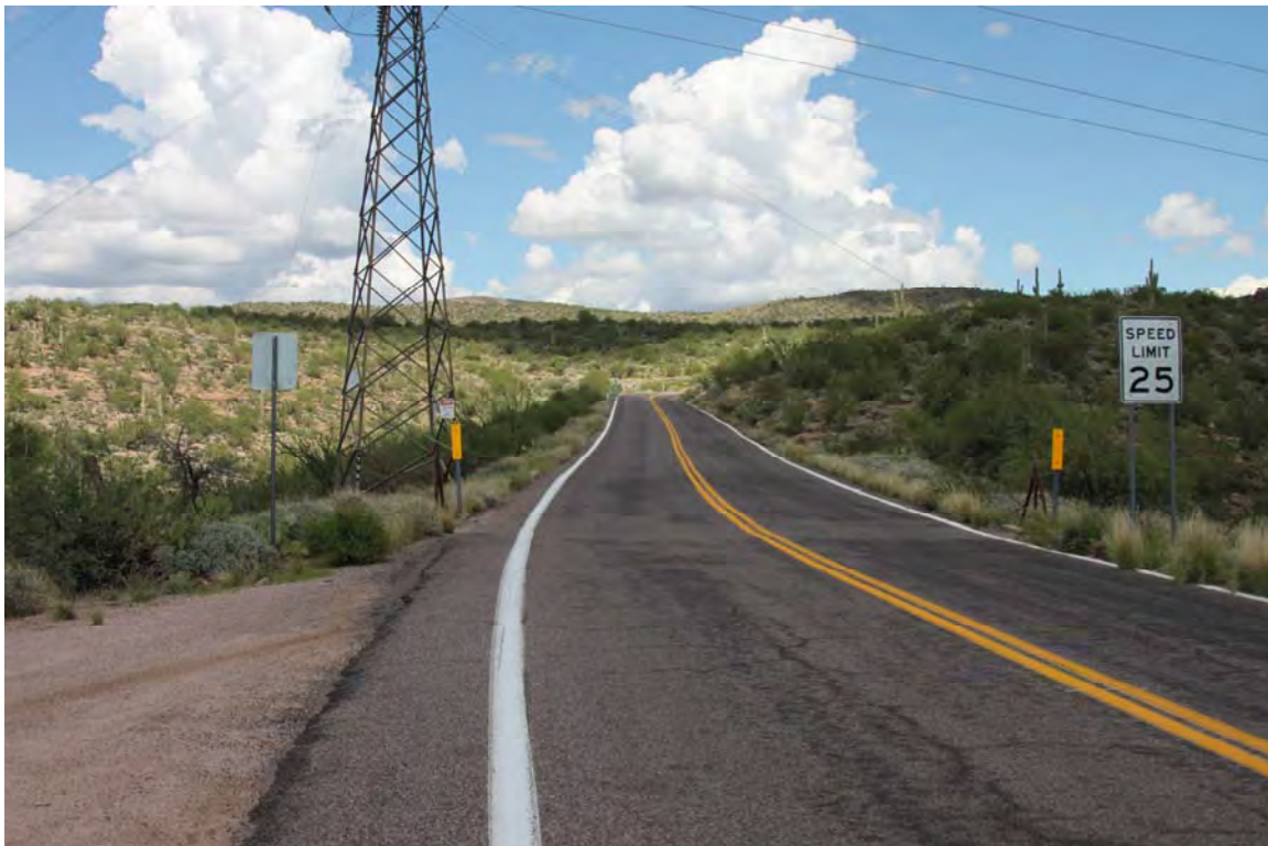
Photo 48. View to the northeast at MP 216.4 (opposite view of the previous photo).
