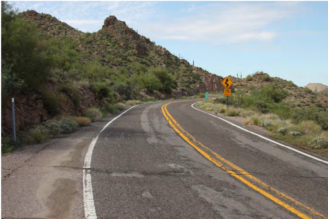
Photo 9. View to the southwest at MP 205.
