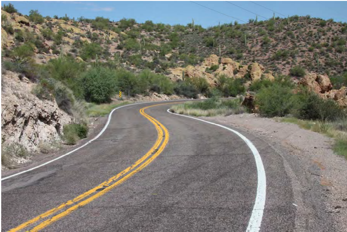
Photo 13. View to the south at MP 207 (opposite view from the previous photo).
