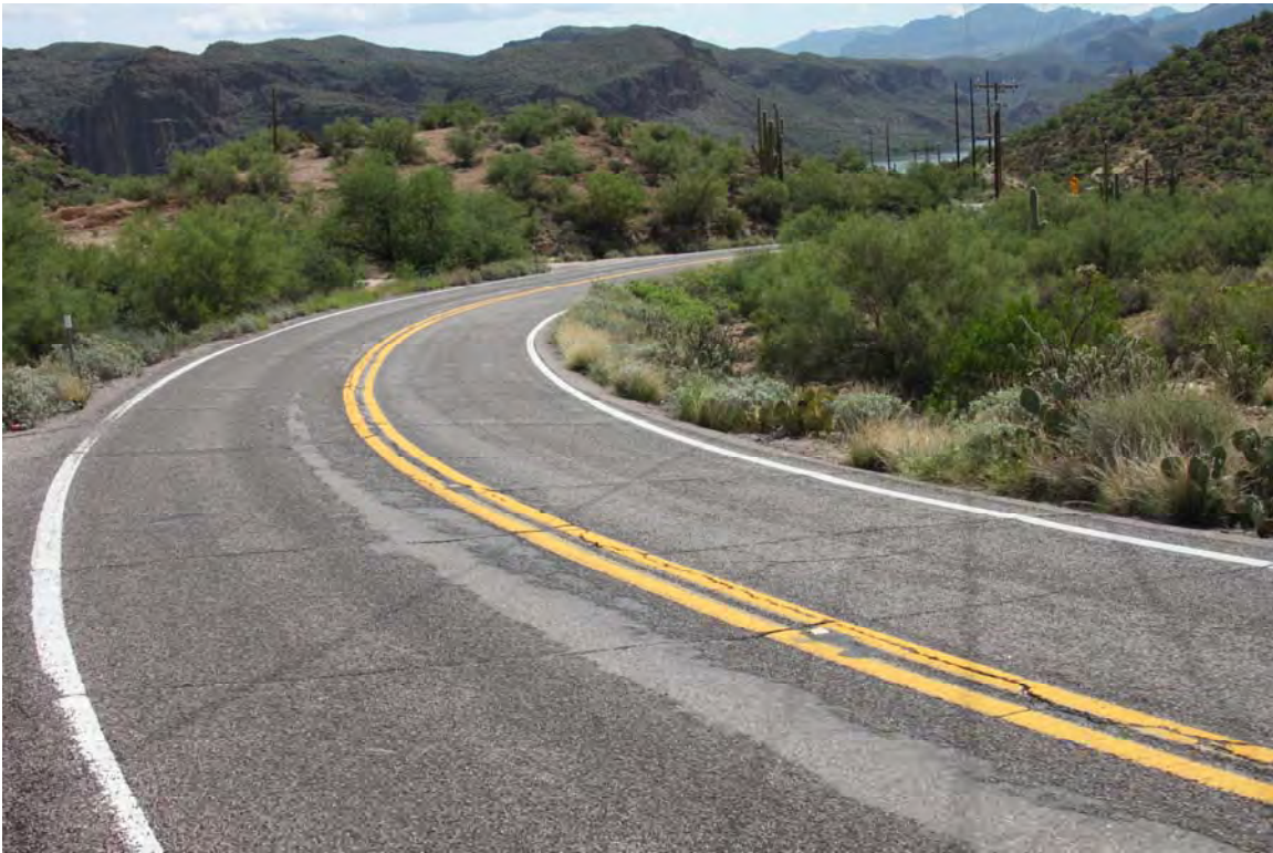
Photo 17. View to the east from the middle of Curve 5 at MP 208.3 (opposite view from the previous photo).
