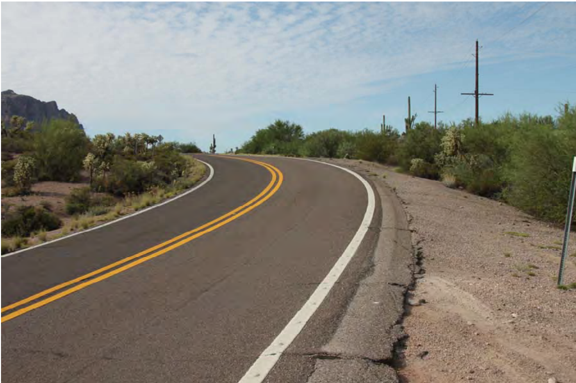
Photo 2. View to the south of Curve 1 at MP 203.5.
