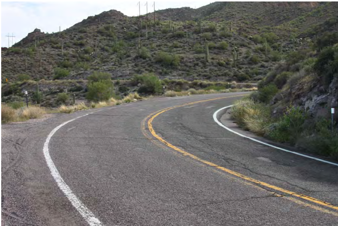
Photo 6. View to the northeast from the middle of Curve 2 at MP 204.3 (opposite view from the previous photo).
