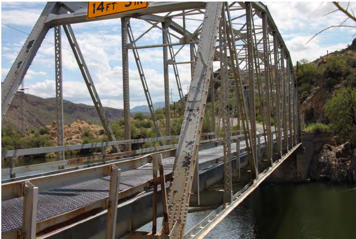
Photo 21. Close-up view of the First Water Creek Bridge.
