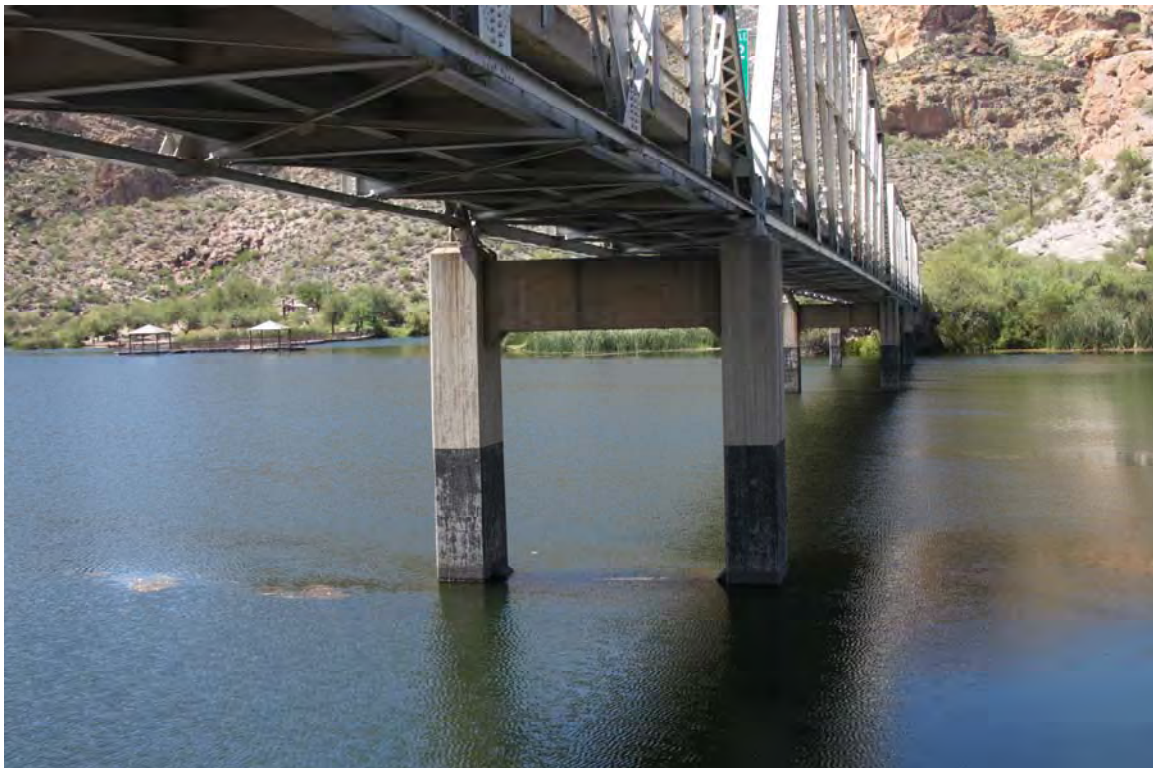
Photo 28. View of the Boulder Canyon Bridge from the eastern bridge abutment.
