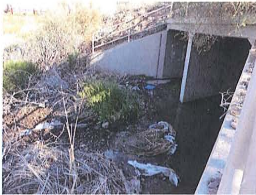
Outfall 101-11.85 with debris present
