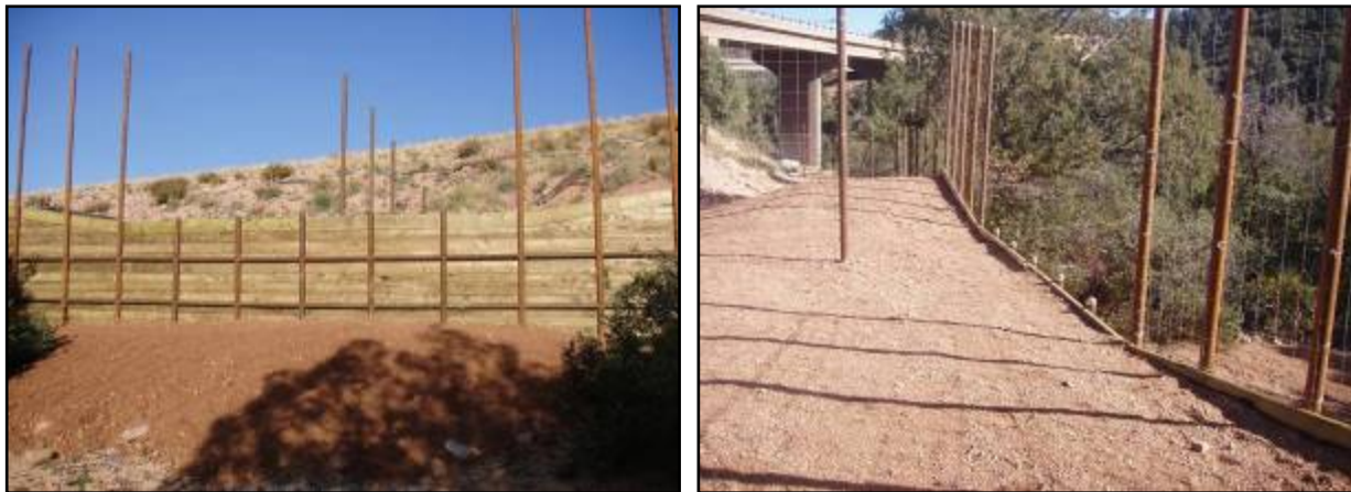
Figure 1. Full-sized in-line wildlife escape ramp with wooden retaining wall constructed on State Route 260. Note the landing pad onto which animals jump off the ramp on the left photo.
