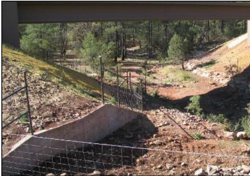
Figure 2. Full-sized in-line wildlife escape ramp with concrete retaining wall constructed on State Route 260. Note the unsuitable rocky substrate at the landing pad below the ramp.
