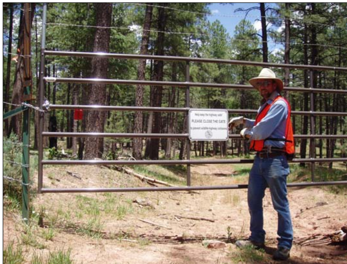
Figure 6. Modified 6-foot Powder River gate installed on a lateral access along State Route 260. Gate was raised to 8 feet with a barbed-wire stinger above the top rail to preclude animals from entering the fenced ROW. Note the sign imploring users to close the gate.
