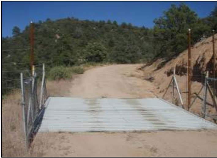
Figure 7. Double-wide cattle guard installed at a lateral access point along State Route 260 to prevent elk encroachment into the fenced ROW.
