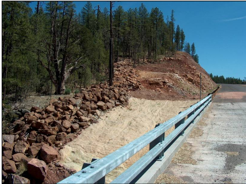
Figure 5. Application of “elk rock” rip-rap in a swath to deter ungulate passage into the highway ROW. In this instance along State Route 260, elk rock was tied into a wildlife underpass.
