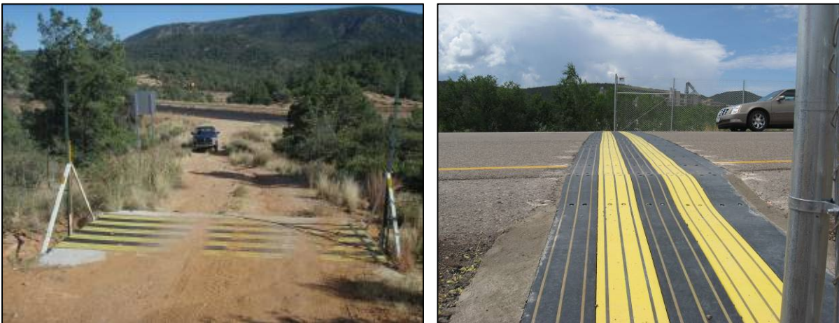
Figure 8. Electrified mats (ElectroMats™) installed along lateral access roads as an alternative to gates and cattle guards on a low volume access road off State Route 260 (left) and an on-ramp on Interstate-40 in New Mexico.
