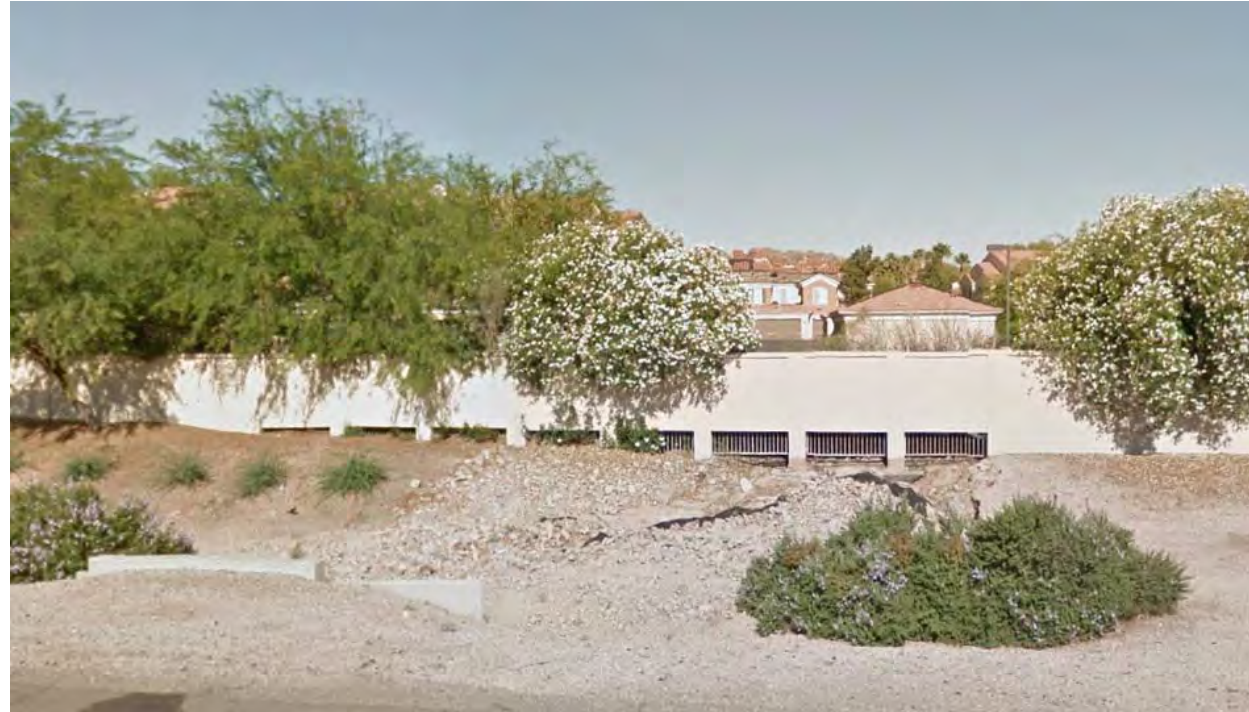
Figure 34 – Existing Drainage Opening in Privacy Wall
