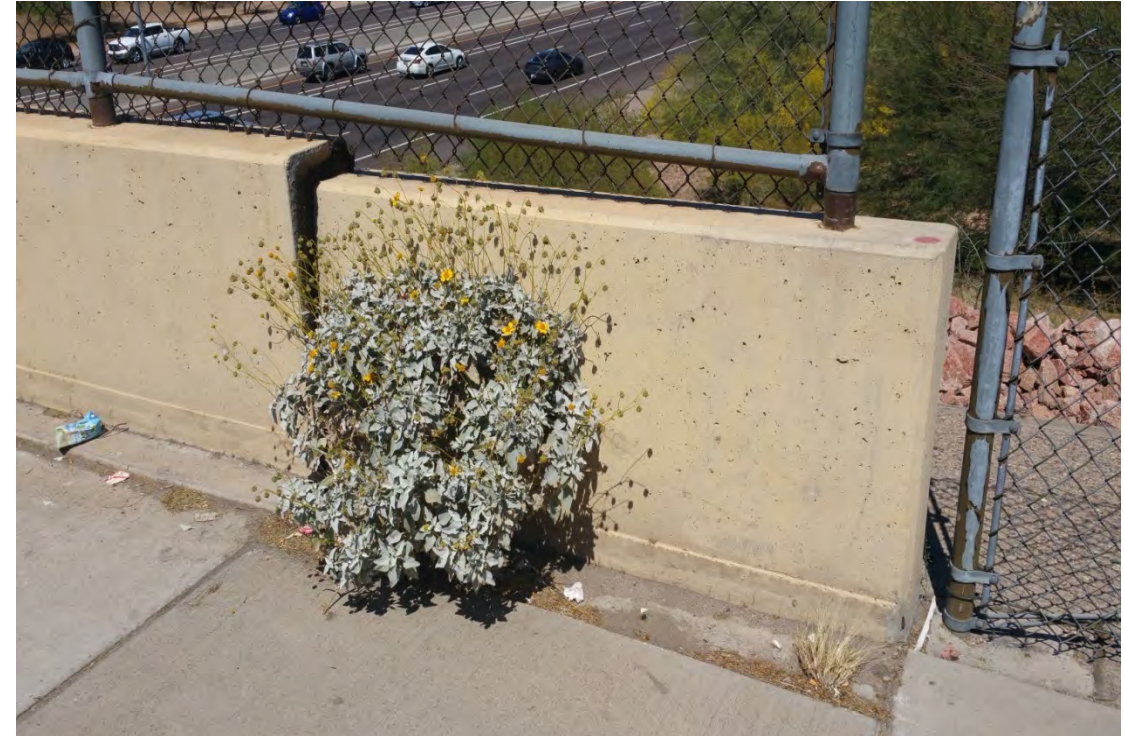
Figure 31 – Elliot Road TI Underpass Fence (Parapet Rotation)
