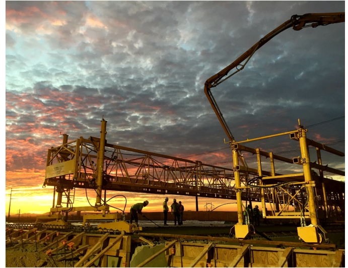
Pouring the 40th Street bridge deck
