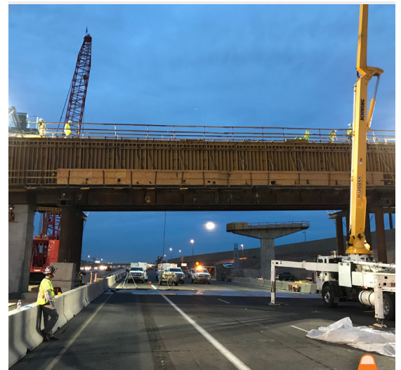
Forming the falsework for a straddle bent over I-10 Papago Freeway
