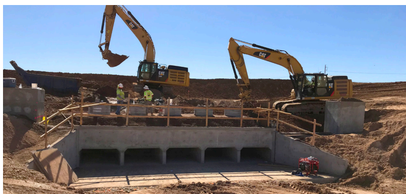
Installing new drainage culvert at Elliot Road
