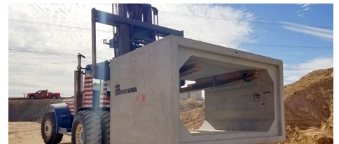
Placing a pre-cast culvert near 24th Street
