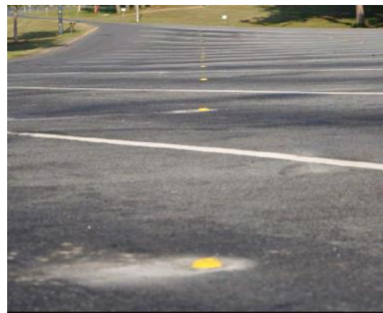
Figure 4-5: Parking Space Occupancy Sensors at a Public Rest Area
