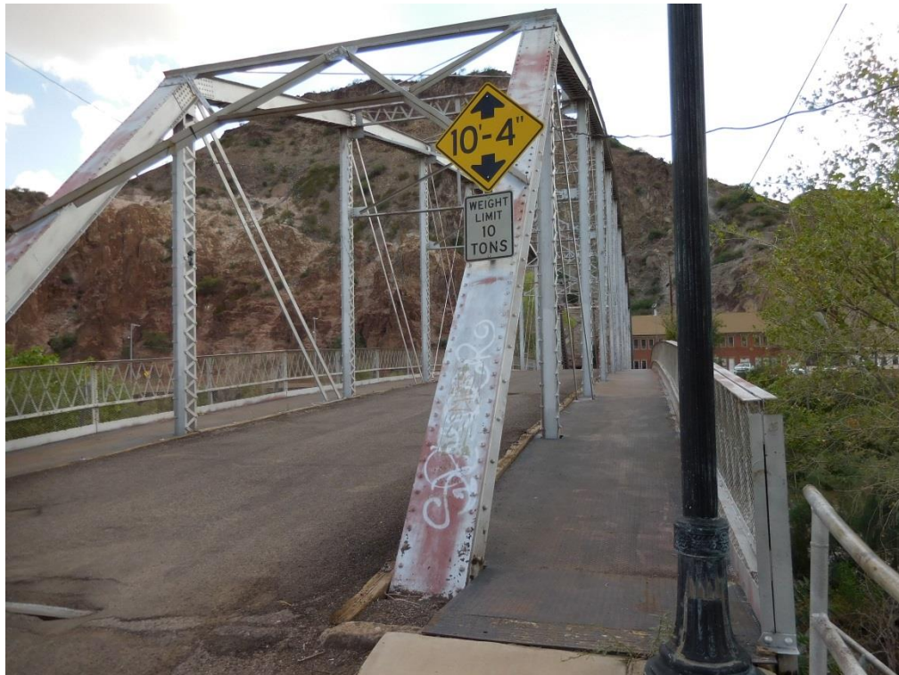
Zorilla Street Bridge – Looking West
