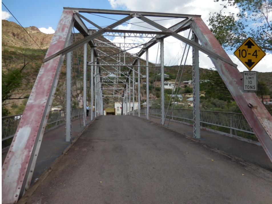
Zorilla Street Bridge – Looking East
