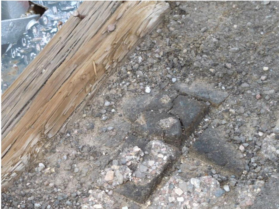
Severed Wood Post Next to Wooden Pavement Edge
