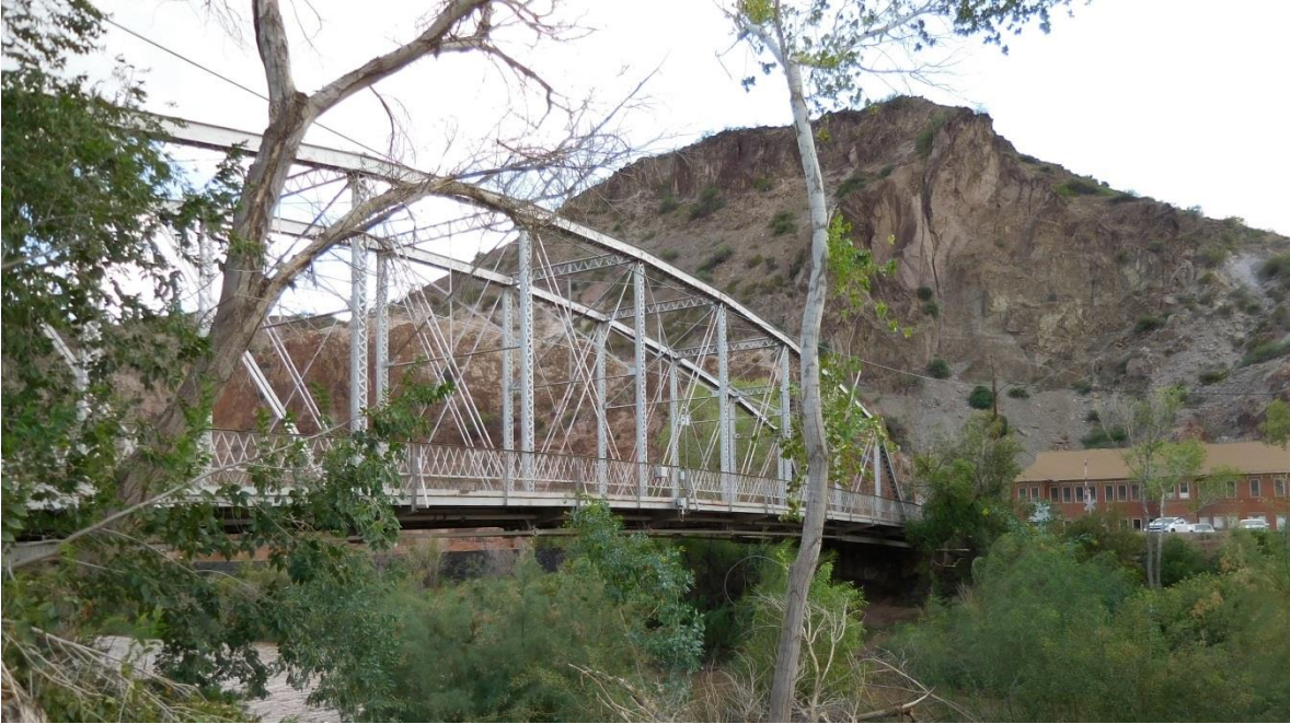
Zorilla Street Bridge – Looking Southwest
