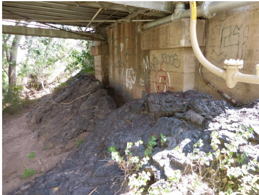
West Abutment – Poured mine slag used as scour protection (Gas main shown)
