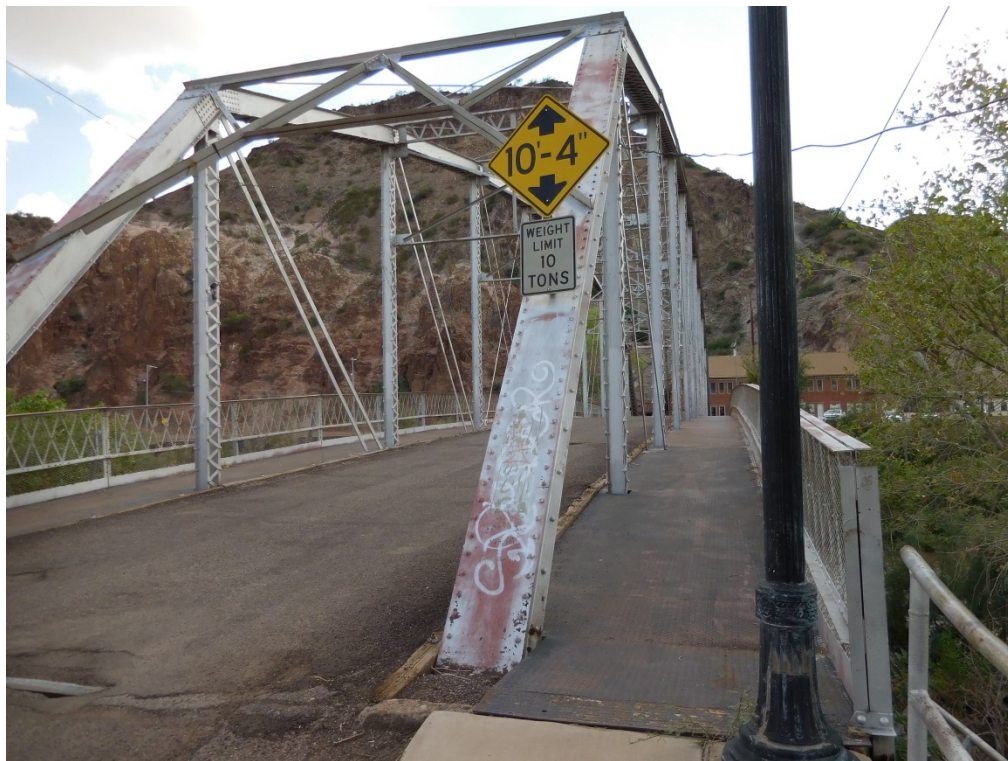
Zorilla Street Bridge – Looking West
