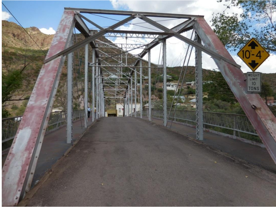
Zorilla Street Bridge – Looking East
