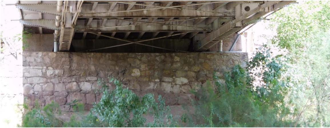
East Abutment – Rock wall built in front of abutment
