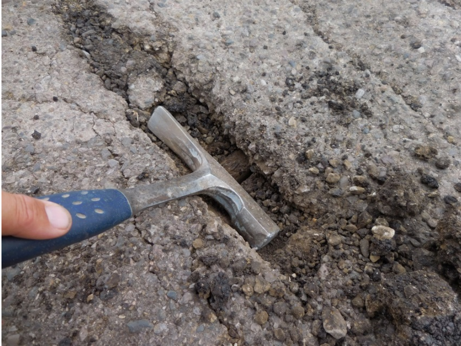
Asphalt Pavement Deck - ~2" Thickness
