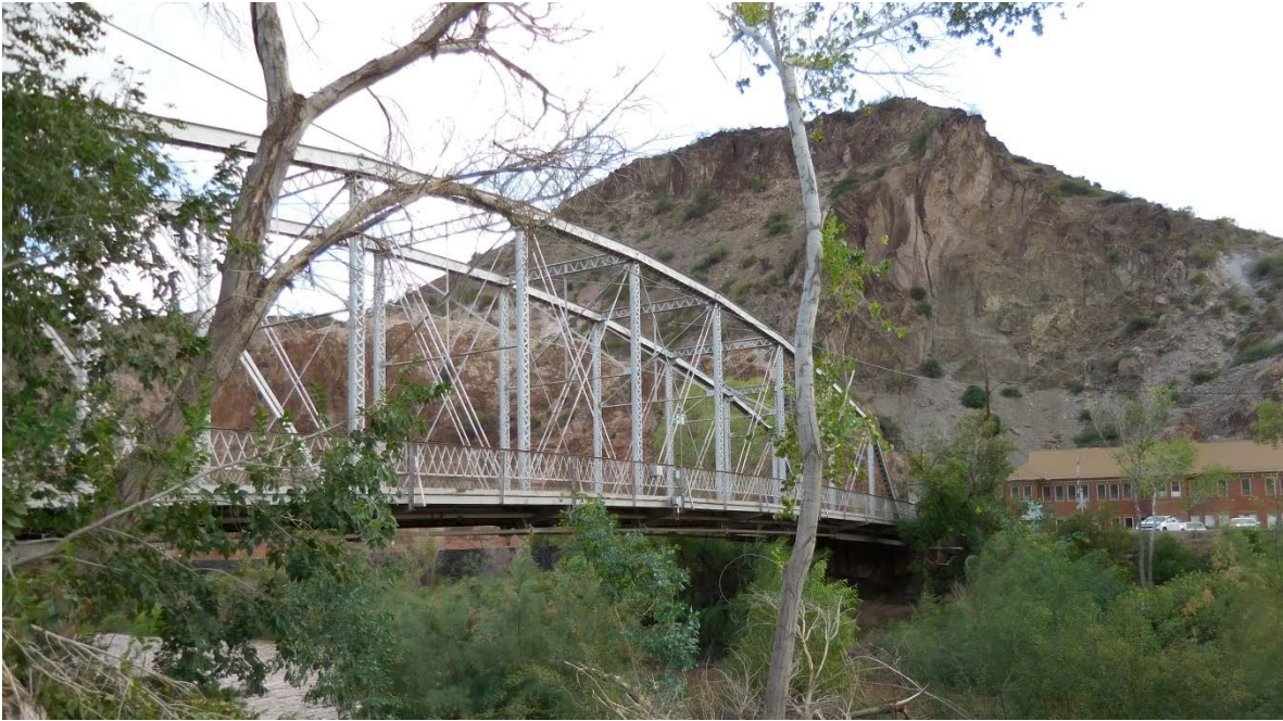
Zorilla Street Bridge – Looking Southwest
