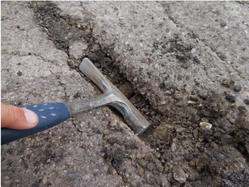
Asphalt Pavement Deck - ~2" Thickness
