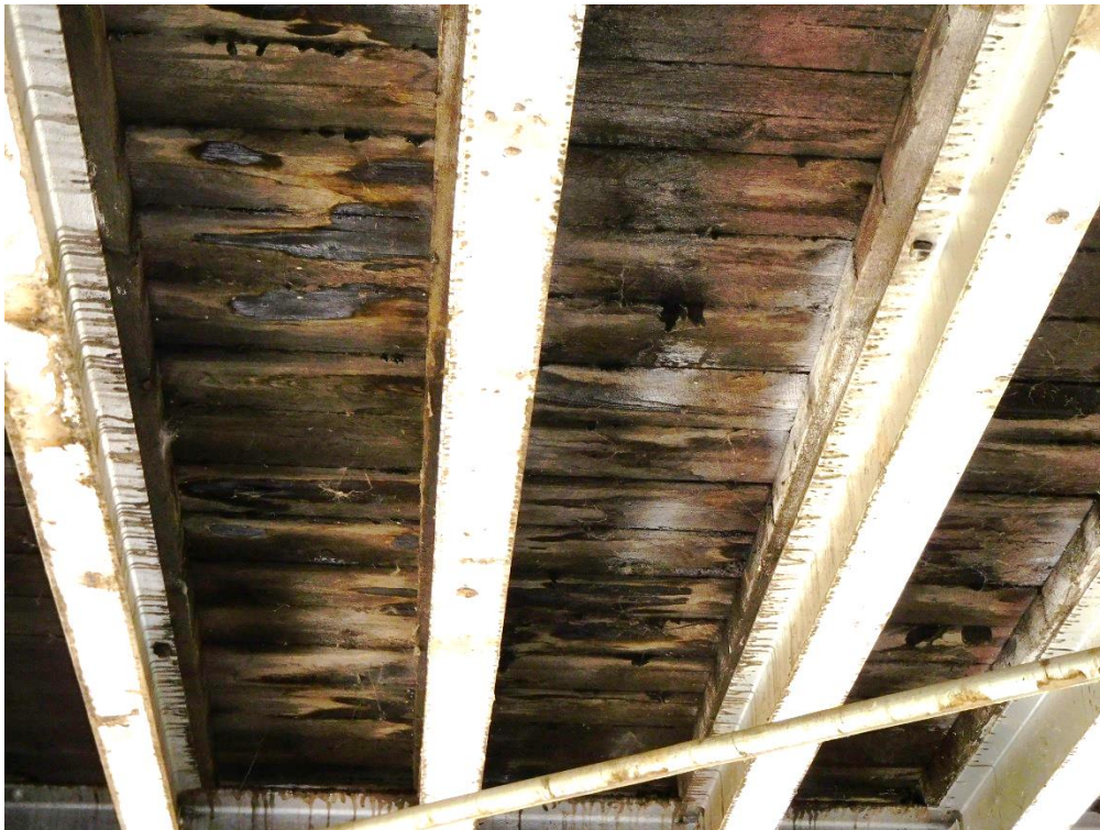
Wood Bridge Deck – Looking up from below
