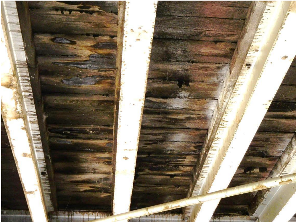
Wood Bridge Deck – Looking up from below
