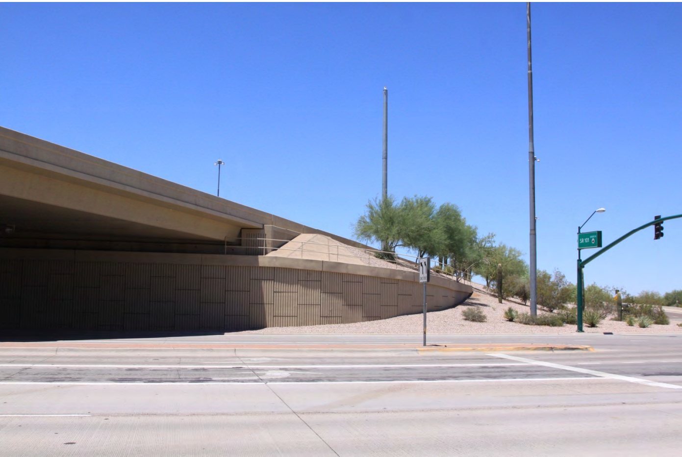
Figure 35 – MSE Walls At 56 th Street Overpass
