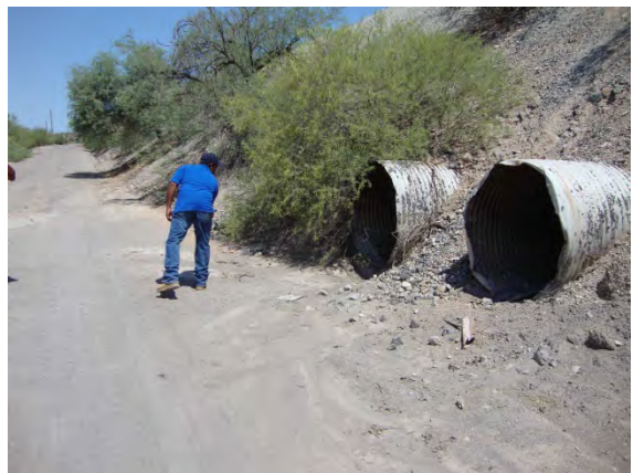
Figure 4 – Two 48-inch CMP
