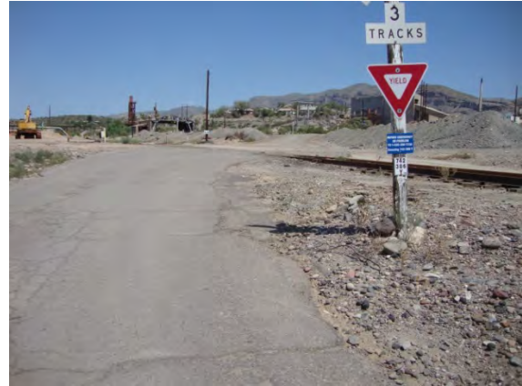
Figure 2 – ASARCO Railroad Crossings
