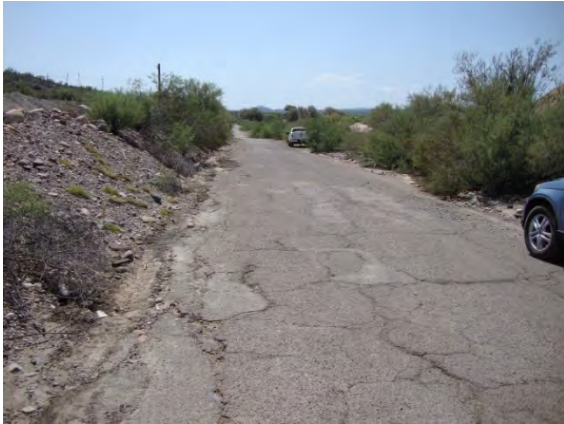
Figure 1 – Cracked Pavement in Hayden
