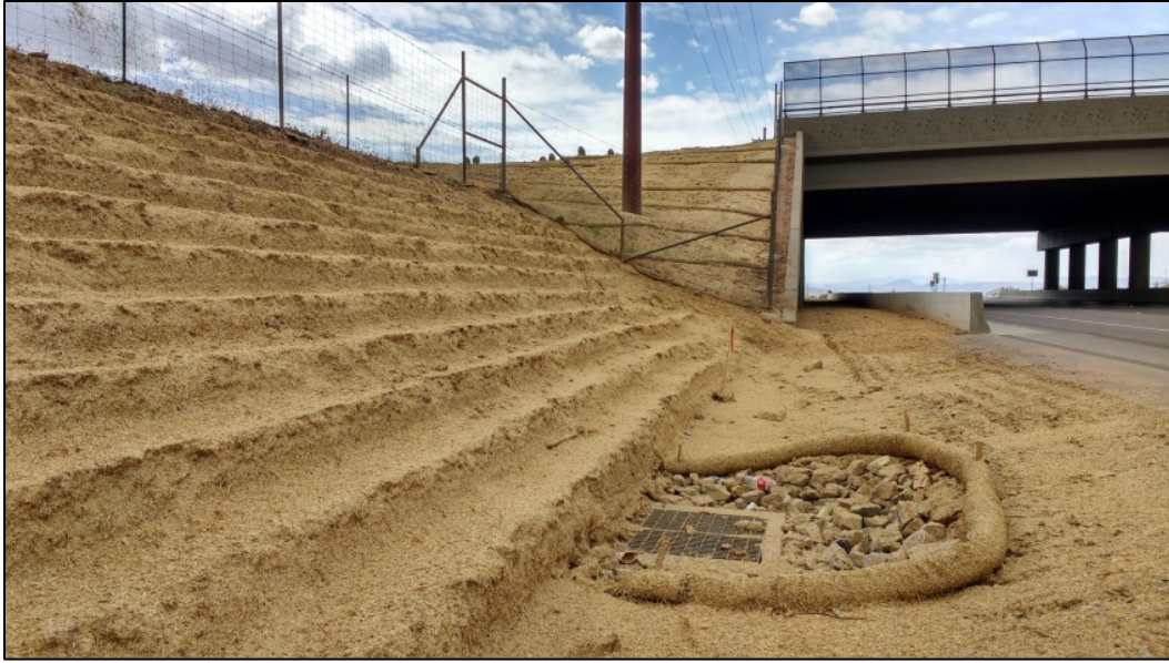
Hydrostraw mulch and tackifier applied to slope
