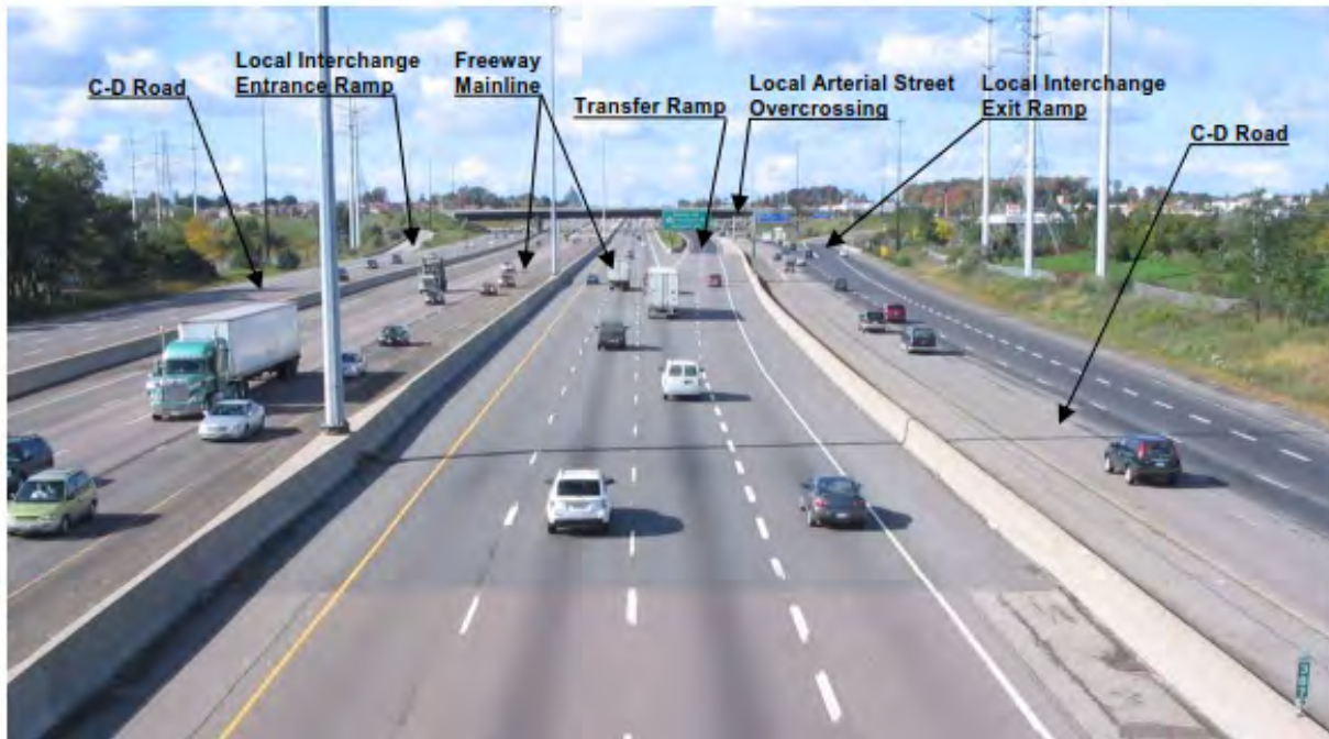
Figure III-2. Freeway with Collector–Distributor Roads
