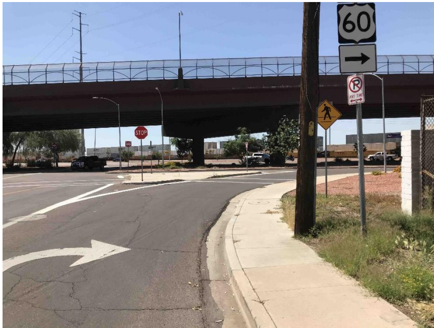
Looking south along 55 th Avenue, subject on the right
