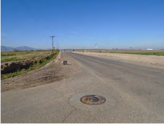
West along Dobbins Road
