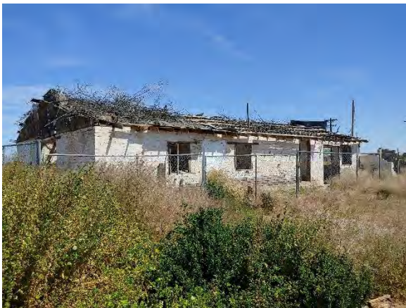
Exterior of Hackin dairy barn
