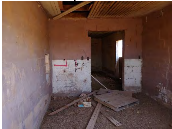
Interior of Barnes dairy barn
