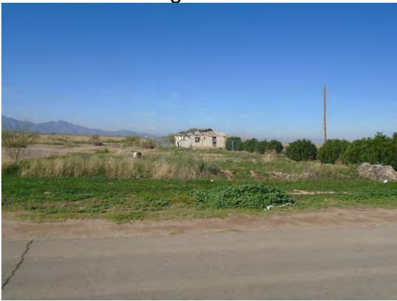
West from 59 th Avenue toward Hackin Dairy Barn
