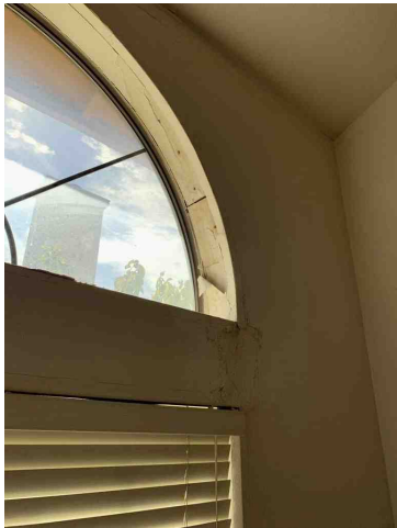
Deferred maintenance - water damage, peeling paint - Living Room
