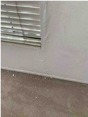
Deferred maintenance - water damage Living Room
