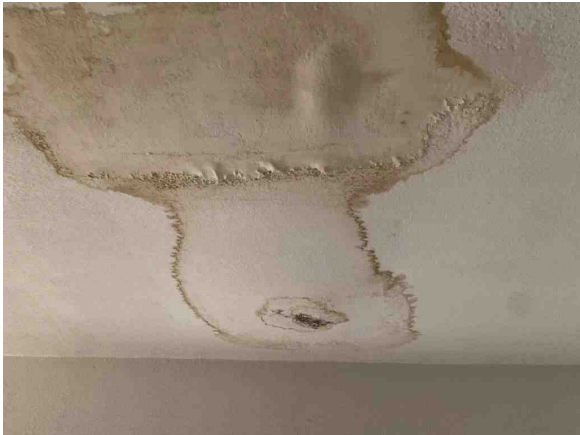
Deferred maintenance - roof leak master bedroom
