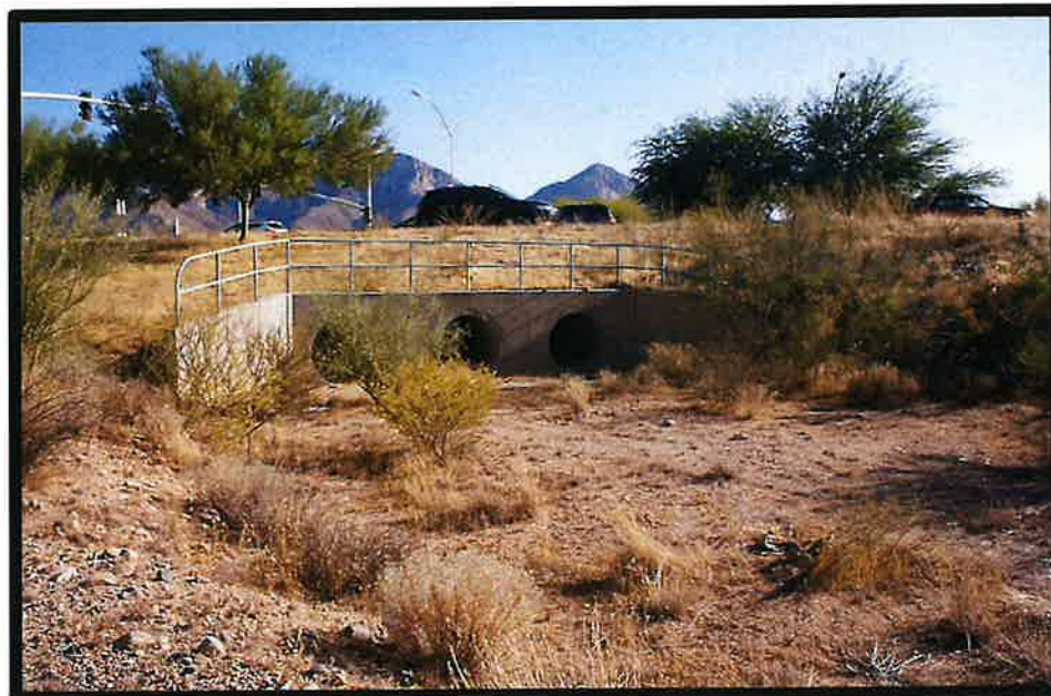
PHOTO 6 – BOX CULVERT IN R/W NEAR SOUTH EAST CORNER
