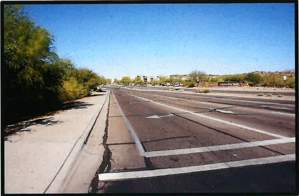
PHOTO 15 – NORTH ALONG INNOVATION
