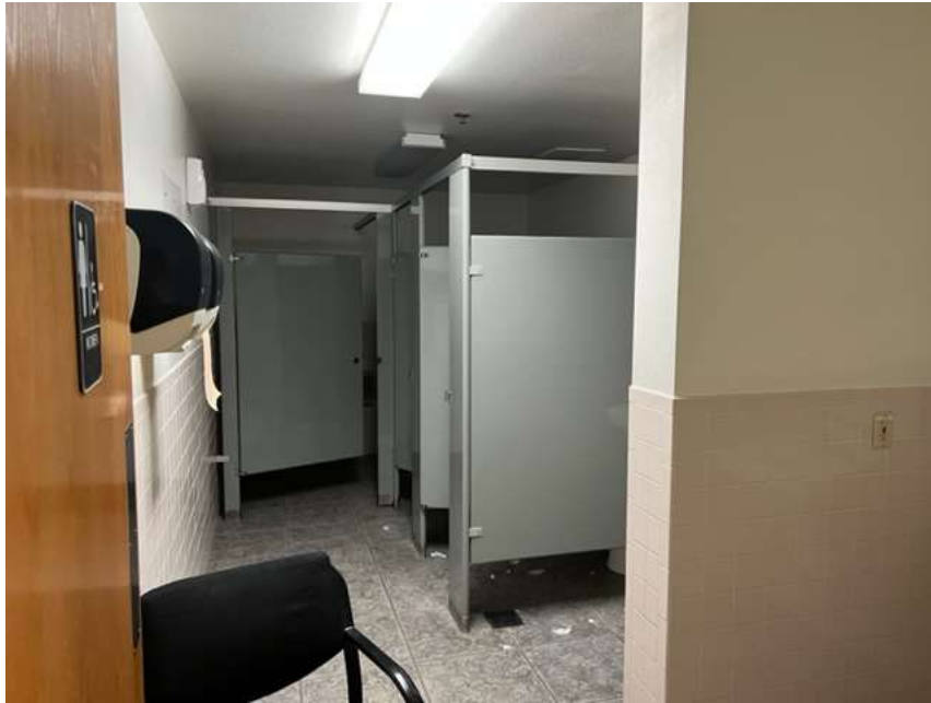
Typical interior of the subject bathroom
