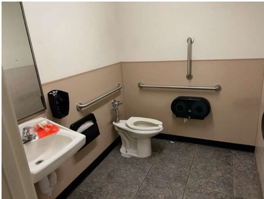
Typical interior of the subject bathroom
