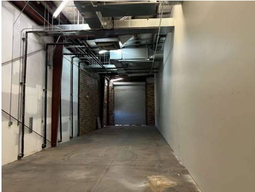
Typical interior of the subject warehouse area in the rear of the building
