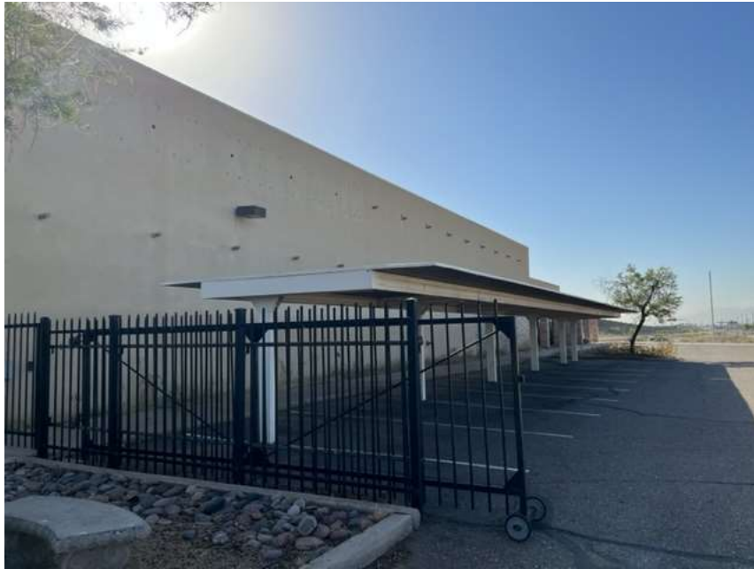
Subject parking area
