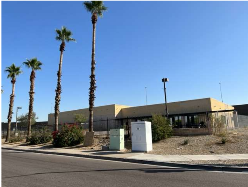
Looking at the exterior of the subject
