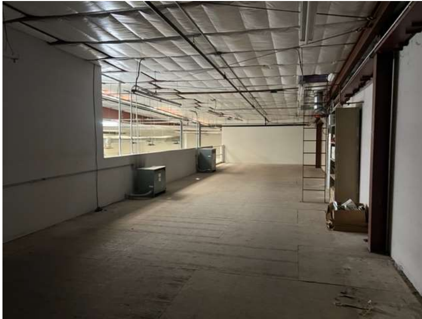
Subject mezzanine area
