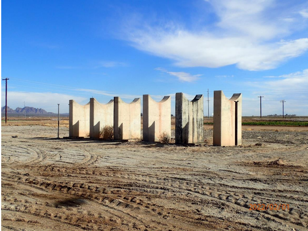
Concrete supports for above ground tank.
