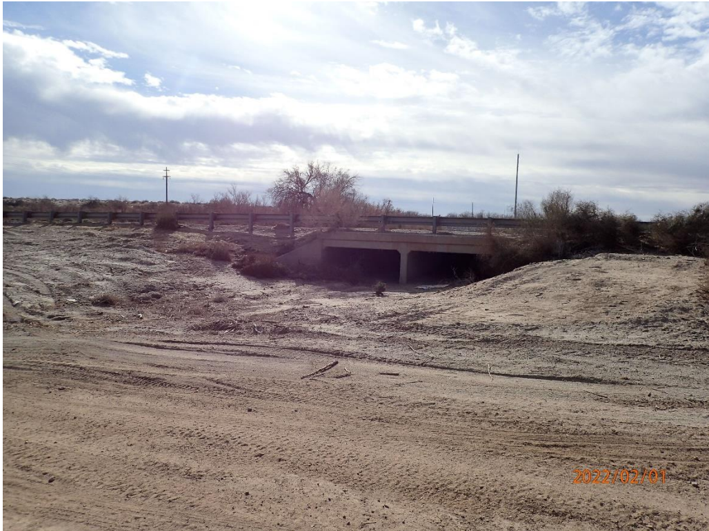
Box culvert under old US Highway 80.
