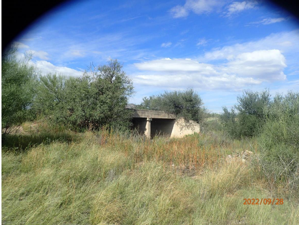
Old bridge in central portion of subject property.
