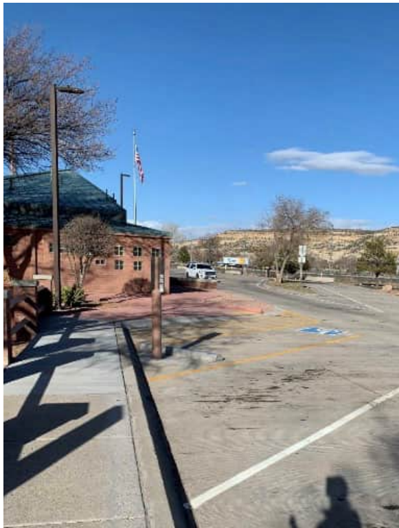
Figure 4-5. ADA Improvements at Rest Areas
