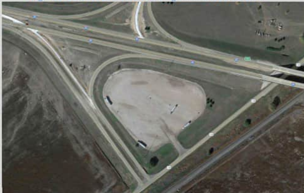
Figure 2-12: Low Cost Truck Parking Solution in Nebraska
