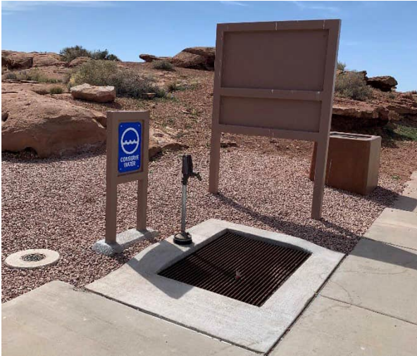
Figure 4-2. Water Conservation Pump, Meteor Crater Rest Area (EB)
