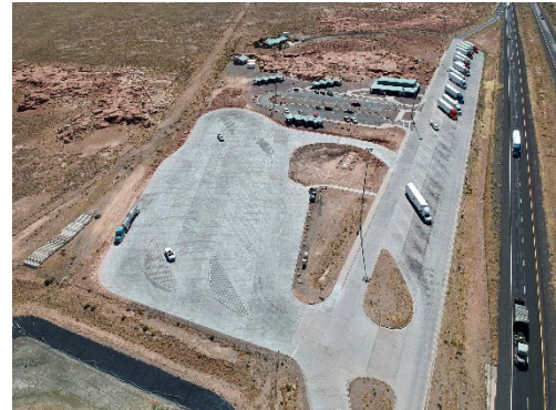
Truck parking expansion at Eastbound Meteor Crater rest area. (Source: ADOT)
