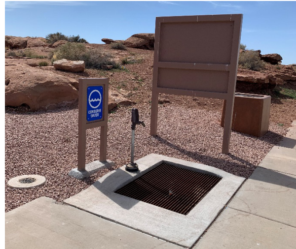
Water Conservation Pump – Meteor Crater Rest Area (EB)
