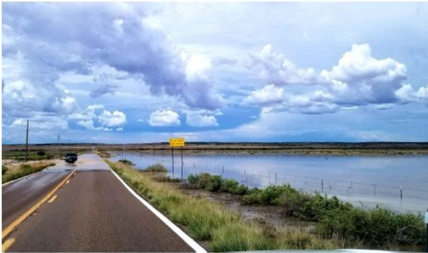
Roadway overtopping at around Sta. 432+00 South of Existing Box Culvert.
