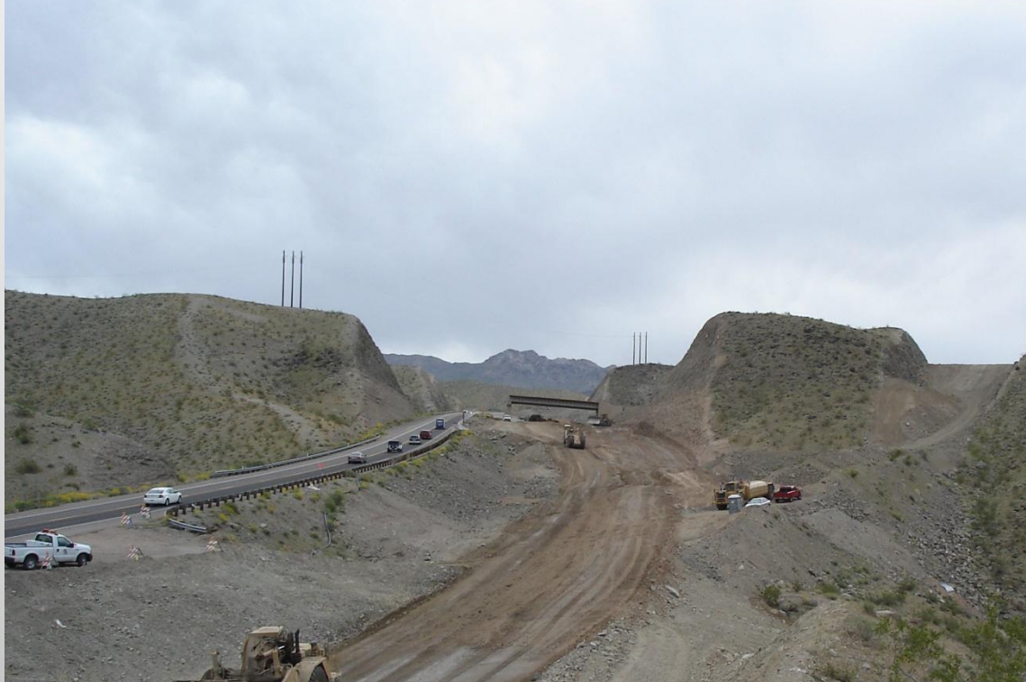
US 93 Two Lanes to Four Lanes
