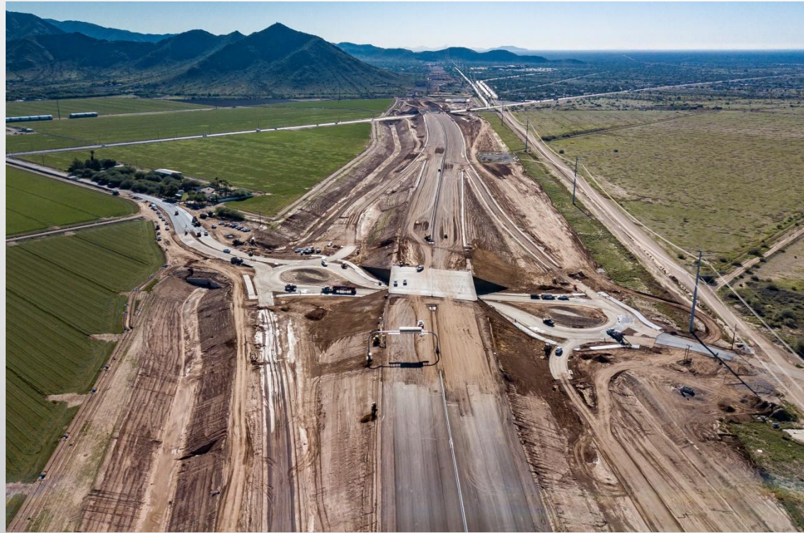
South Mountain Freeway
