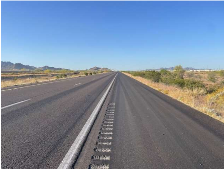
South on State Route 85
