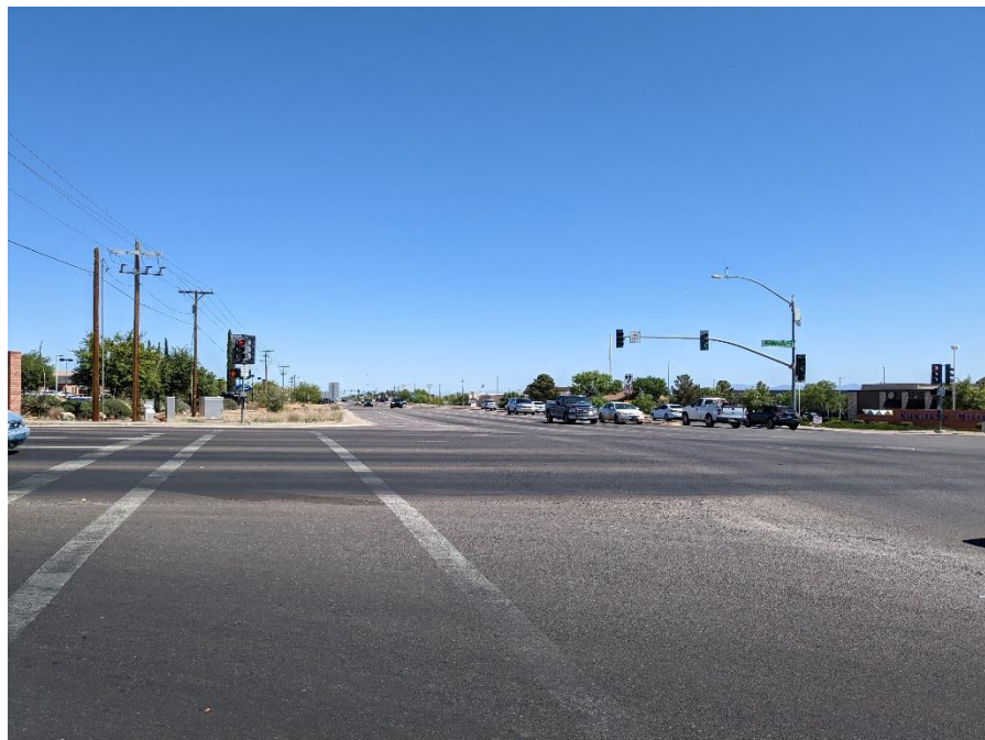
Hy 90/Hy 92 intersection looking north
