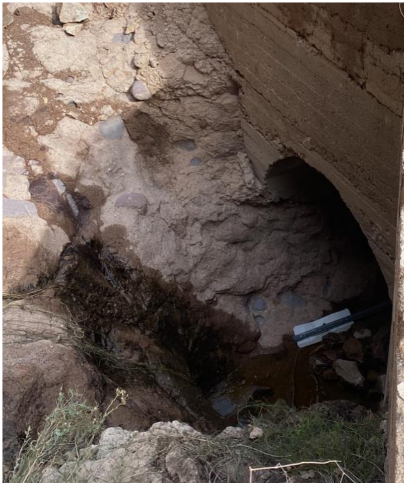
Photograph 14. One of the many concrete structures observed.
