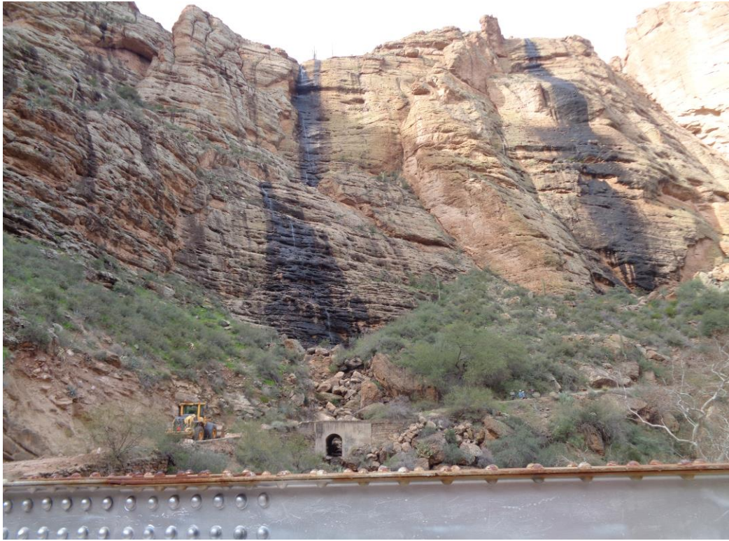
Photograph 7. View facing west from the Fish Creek Bridge.
