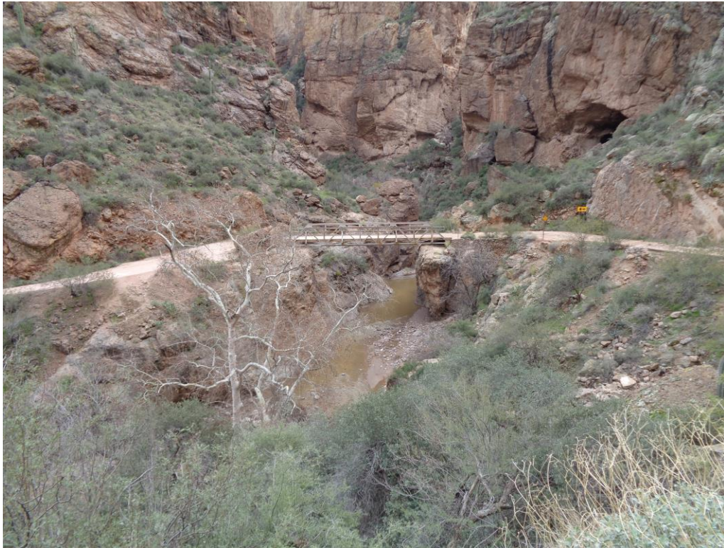
Photograph 3. Overview of the Fish Creek bridge at MP 223.5.
