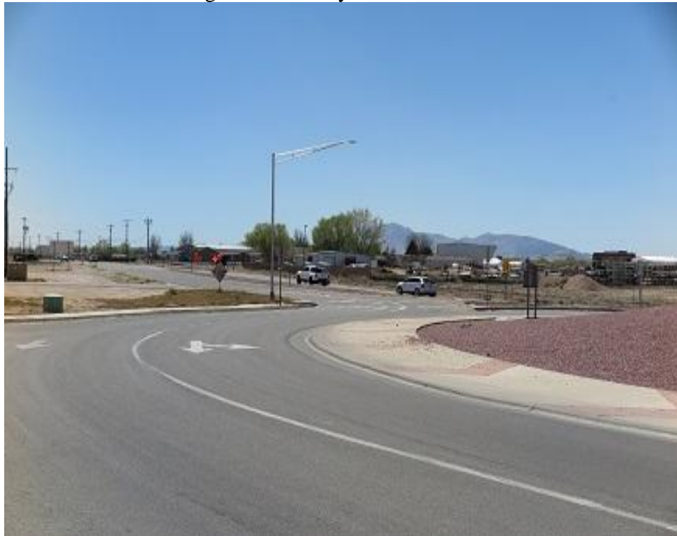
Street View – Looking Southwesterly SR 89 and RD 4 North Roundabout
