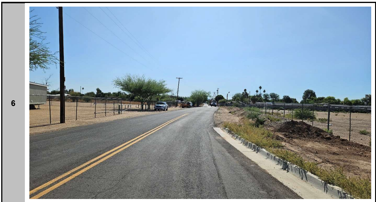
View east along Orangewood Avenue at Grand Avenue (US Highway 60)
