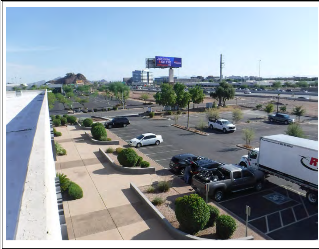
EAST SIDE PROPERTY VIEWS, FROM THE SUBJECT PROPERTY BUILDING ROOF
