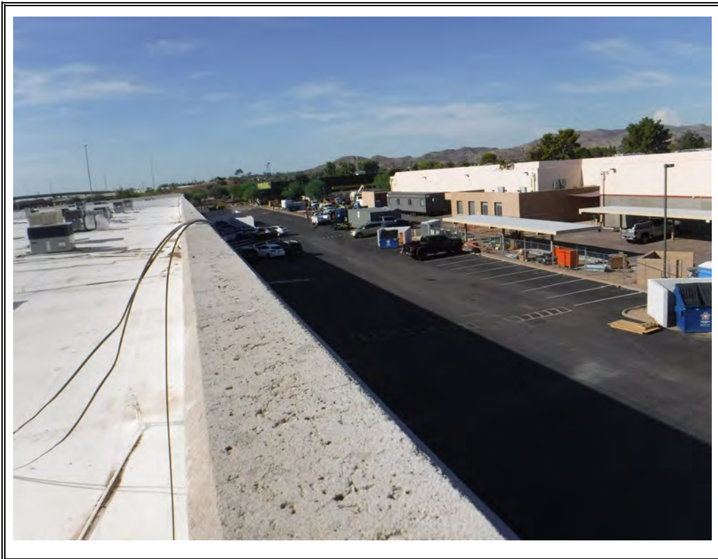
WEST REAR PROPERTY VIEW FROM THE ROOF
