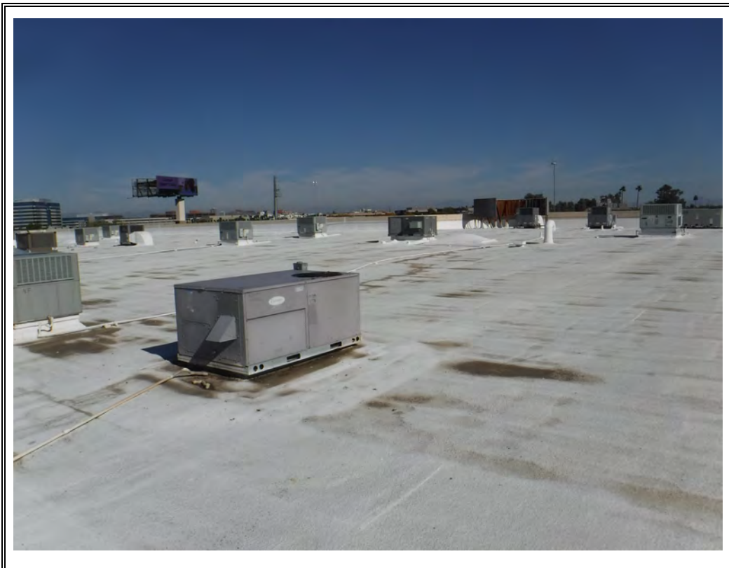
ROOF VIEW OVER SUITES 1-4
