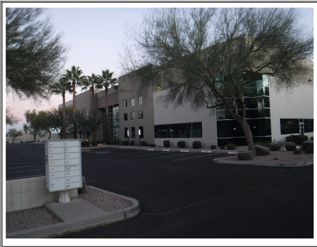
6825 WEST GALVESTION STREET, CHANDLER
