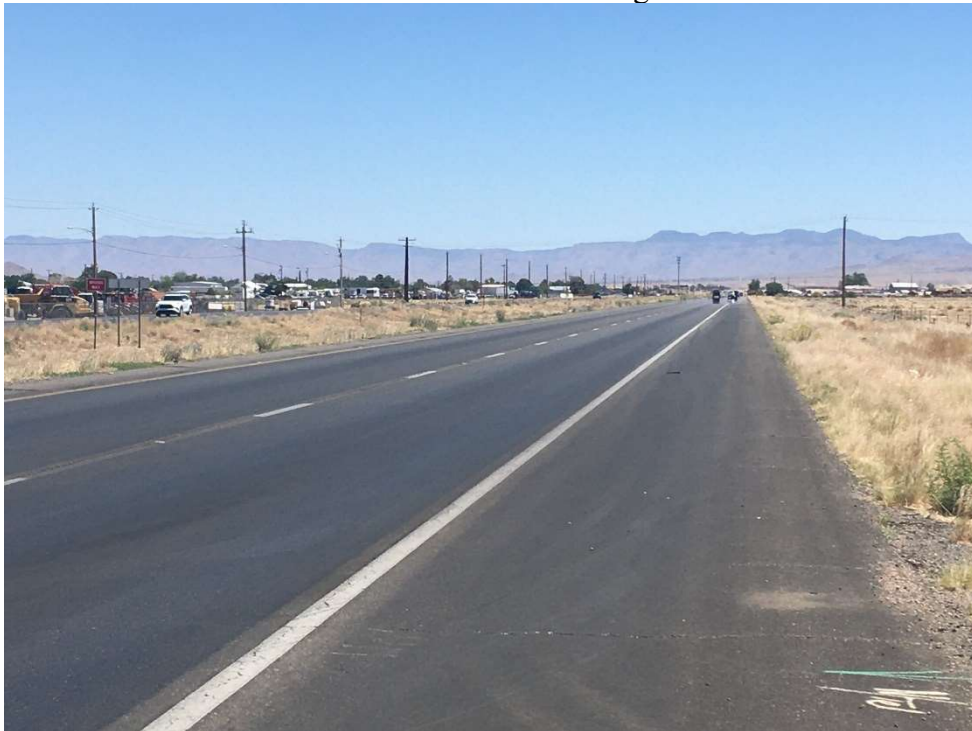
Street View – SR 66 looking NE
