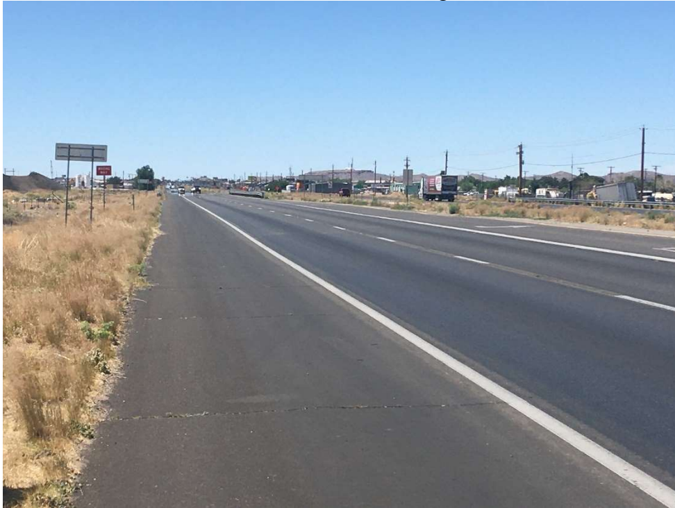
Street View – SR 66 looking SW
