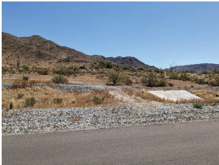
Western potential point of access (just left of concrete) (172323563)
