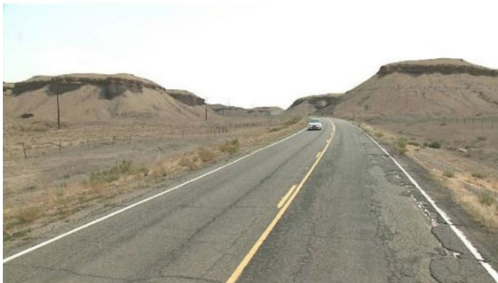
Typical Section of ITHMAS Corridor Showing Poor Quality of Pavement and Narrow Shoulders
