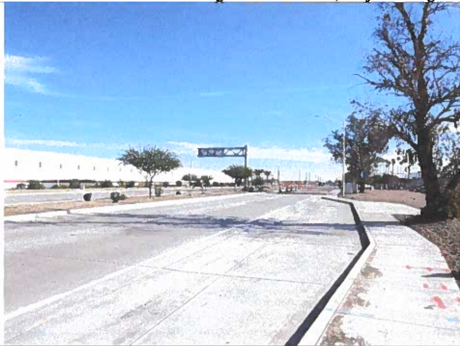
Photo 6: Street View East Along Van Buren Street, Subject on Right
