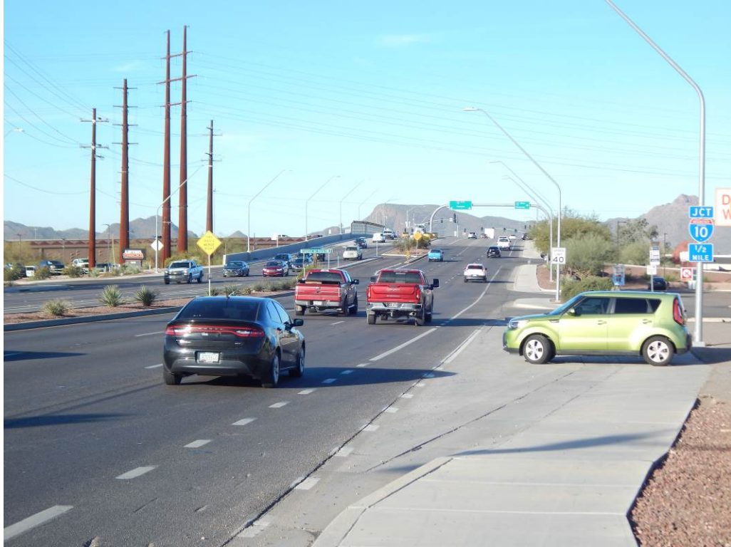
Street View – Ina Road facing west
