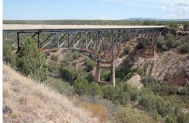
Bridge projects normally are processed with a CE.
