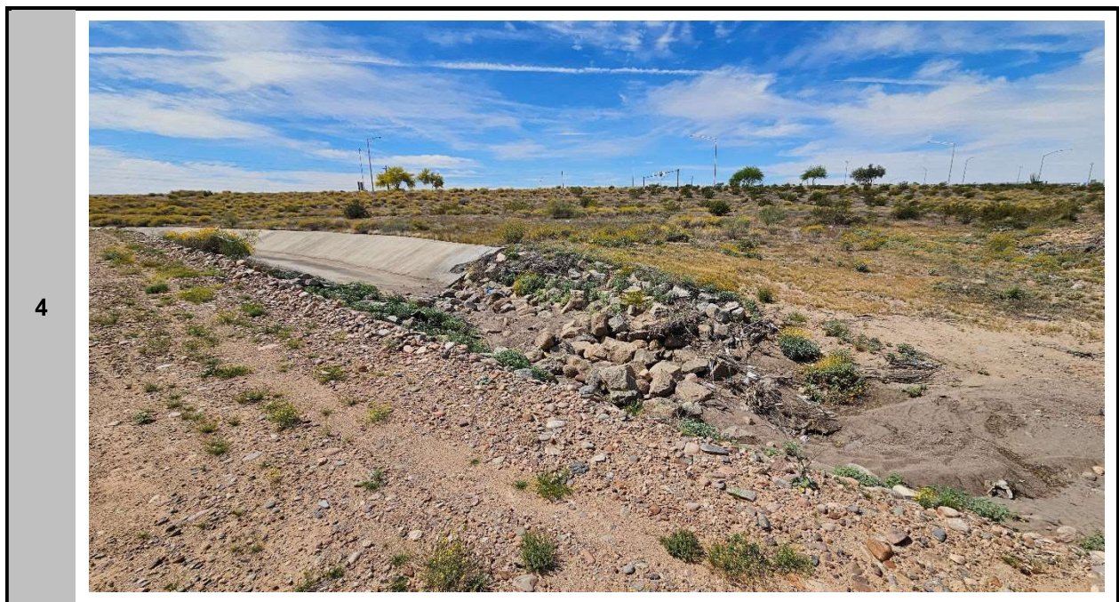
View south across drainage channel
