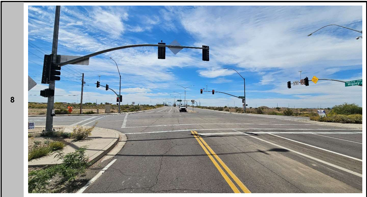
View south along Higley Road at Thomas Road
