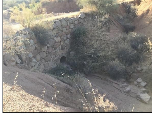
Figure 7. Highly visible culvert headwall prior to flood damage
